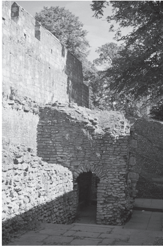
Figure 20 Tower 19 (the ‘Anglian Tower’) in the fortifications of York. The Roman wall here is that of the legionary fortress, robbed of its outer skin in later times so that only the rubble core is preserved. This was covered by the ninth-century defensive bank, on top of which the medieval city walls were constructed. The bank is visible behind the ‘Anglian Tower’ but it has been stripped away by archaeologists to reveal the Roman wall. The ‘Anglian Tower’ seems to plug what was a breach in the Roman wall. Its masonry was clearly quite different from the Roman masonry, which would have been of large square blocks called ashlar, and the voussoirs (i.e. the radiating stones) around its doorway suggest the possibility that it is of seventh- or eighth-century date.
