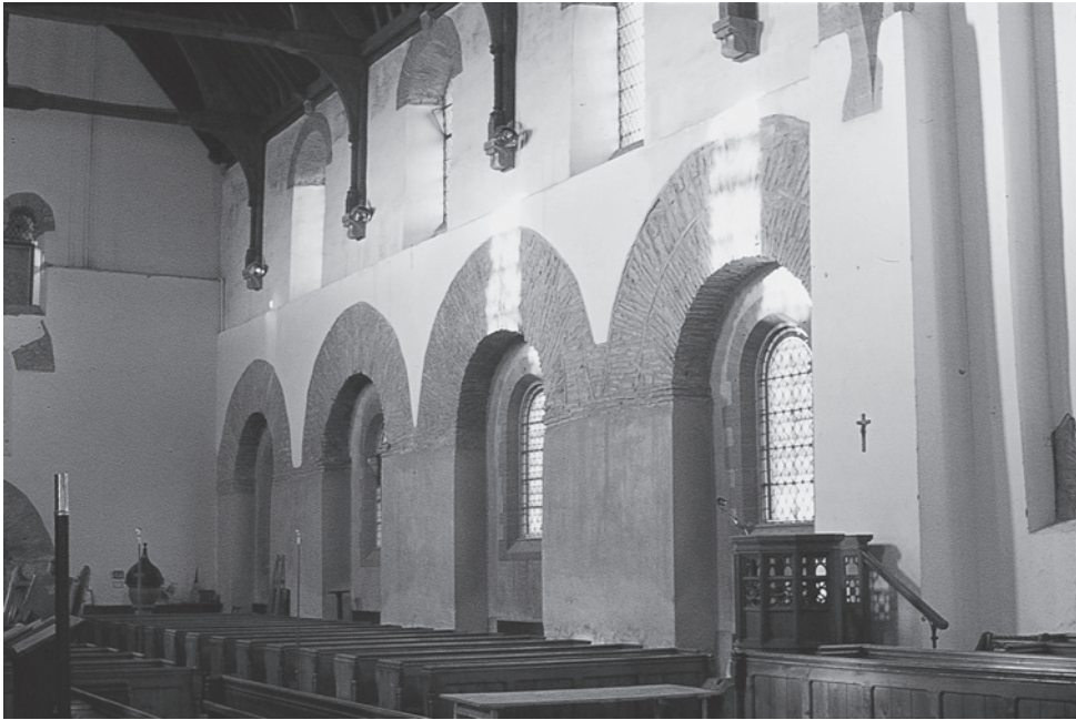
Figure 32 The nave of Brixworth church (Northamptonshire), interior looking west. The large arches to either side would originally have opened into lines of side-chapels or porticus . Notice how Roman they are in style with their radiating lines of tiles, and notice too the rectangular shape of the church itself, which (when still complete) would have resembled a Roman basilica, but one with aisles to either side of the central nave.
