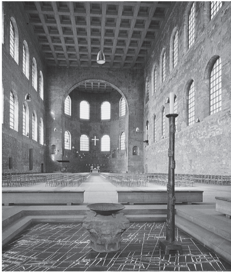
Figure 31 Interior of the Roman basilica at Trier (Germany). Although this building has been much restored and is now used as a church, the basic form and scale of the Roman architecture is still clearly evident. The lines of round windows are original in form, as the masonry on the exterior demonstrates. Notice the rectangular shape of the basilica, with the great arch opening into the semi-circular apse, or termination of the building, where the emperor would have sat to preside over meetings and trials.
