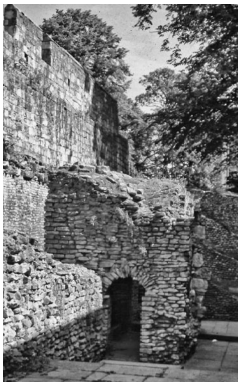
Figure 11.1 Tower 19 (the 'Anglian Tower') in the fortifications of York. The Roman wall here is that of the legionary fortress, robbed of its outer skin in later times so that only the rubble core is preserved. This was covered by the ninth-century defensive bank, on top of which the medieval city walls were constructed. The bank is visible behind the 'Anglian Tower' but it has been stripped away by archaeologists to reveal the Roman wall. The 'Anglian Tower' seems to plug what was a breach in the Roman wall. Its masonry was clearly quite different from the Roman masonry, which would have been of large square blocks called ashlar, and the voussoirs (i.e. the radiating stones) around its doorway suggest the possibility that it is of seventh- or eighth-century date.
