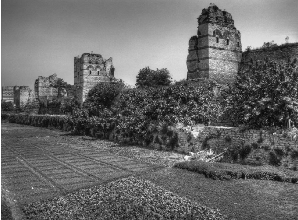
Figure 3.3 The land-walls of Constantinople. In the foreground is the moat. Notice the remains of the breastwork (or wall) on its inner side, with a terrace behind that, itself backed by the remains of the outer wall. Behind it was another space, which an enemy would have to cross under fire, and behind that again was the inner wall, lined with flanking towers, from which the defenders could fire missiles.
