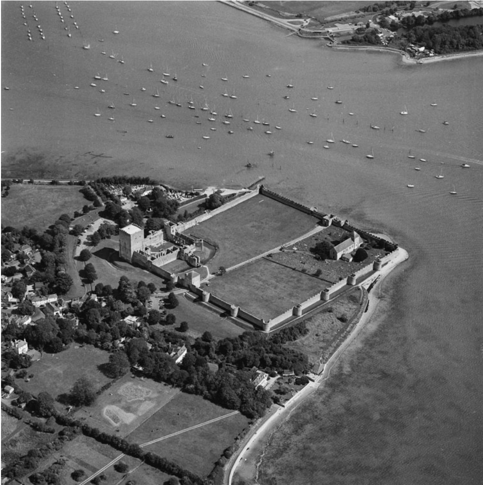
Figure 2.1 Portchester Saxon Shore fort from the air. The wall surrounding the fort is 10ft thick and over 20ft high. The rectangular structure in the top left-hand corner is a medieval castle which was built to make use of a small part of the surviving Roman walls.
