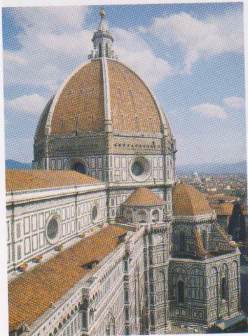
Filippo Brunelleschi's great dome at the cathedral of Santa Maria del Fiore in Florence. Completed in 1436, the dome – the largest ever constructed in bricks and mortar – is one of the outstanding achievements of Renaissance architecture. Its size reflected Florentine determination to excel in all things.
