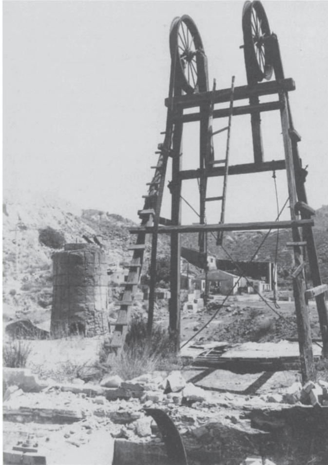
Figure 29.10 The derelict headstocks and calcining furnace on the Cruz Chicita mine in the Murcian mining field of south-eastern Spain. Photograph: M.Palmer.
