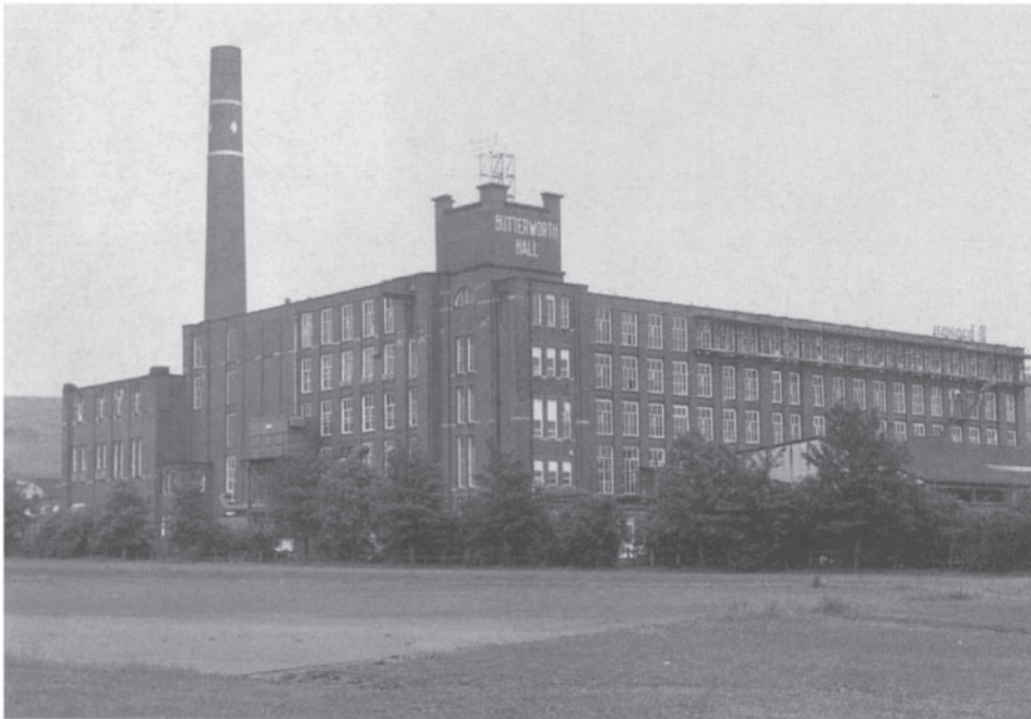
Figure 29.2 Standardization: one of the many cotton spinning mills built in Lancashire, England, using Accrington brick. The only concession to individualism is the name of the company on the corner tower housing the water sprinkler cistern. Photograph: M.Palmer.
