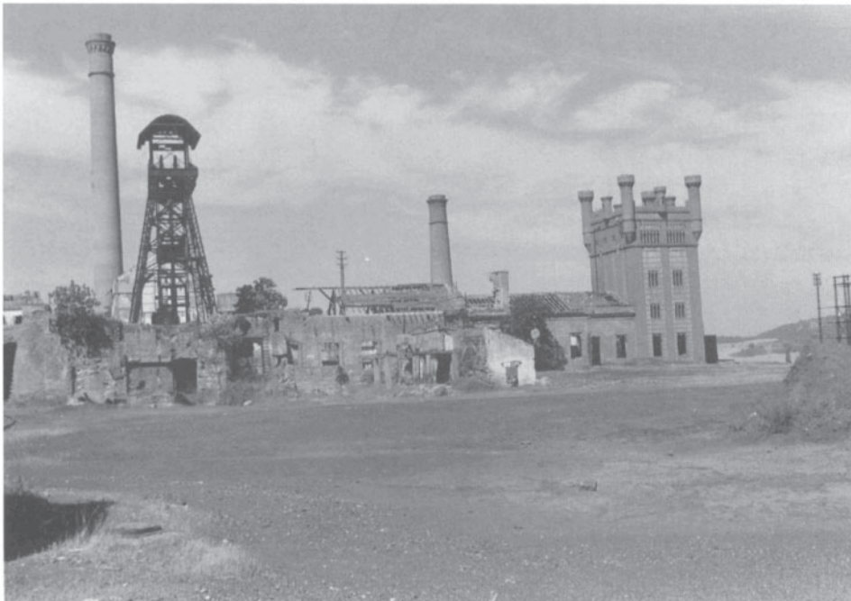
Figure 29.3 Individualism displayed on a coal-mining complex in southern Spain. The functional pit head structures contrast with the bartizan-bedecked electricity transformer house on the right. Photograph: M.Palmer.
