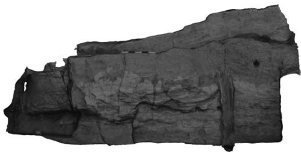
Figure 12. Orthophoto of B.97 south wall section generated using image-based 3D modelling.
