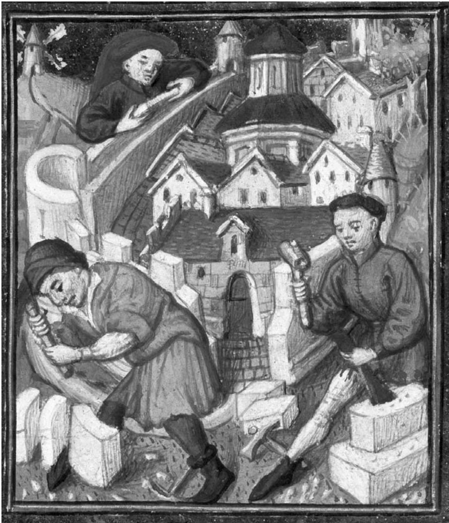
A 15th-century artist represented the importance of stone by showing masons towering over their building project. Each is working with typical masons' tools on a different phase of cutting, shaping, and placing blocks. In the far upper left corner, there is a windmill against the horizon. (The British Library/StockphotoPro)
