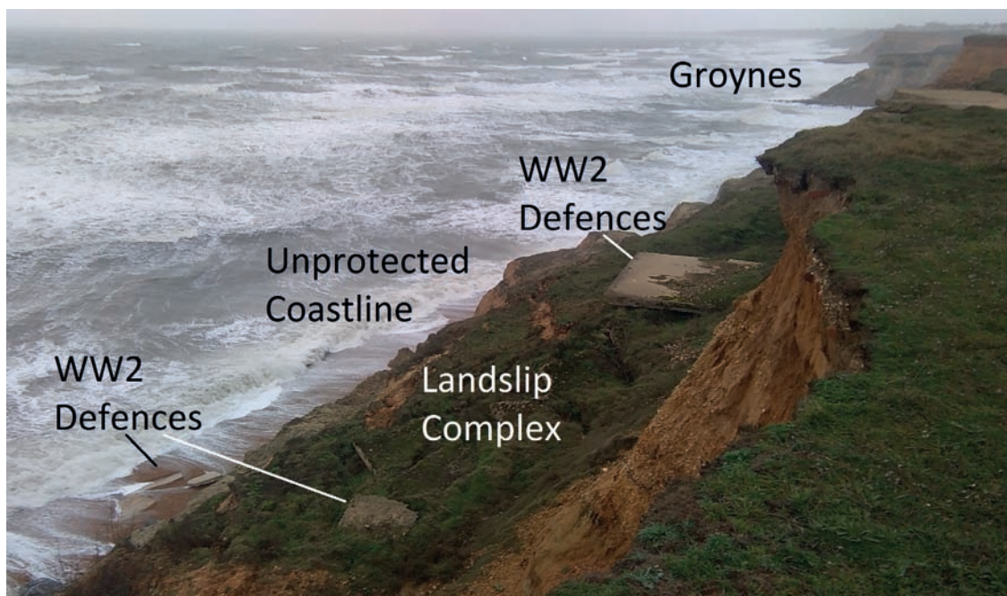
Figure 4.2. Unprotected cliff at Barton-on-Sea, Hampshire, UK, showing the loss of WW2 heritage sites. The Dorset seafront to the east is protected by groynes where the cliffs have stabilised (Photo: G. Momber; MAT).
