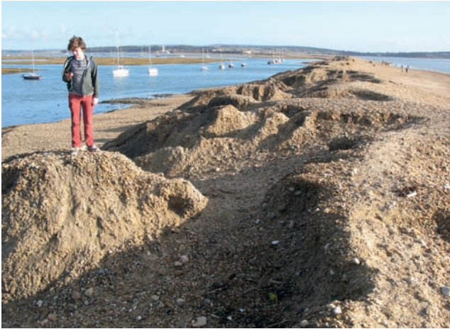
Figure 4.4. Hurst Spit, Hampshire, UK, is breached in the winter of 2015. It was quickly reconstructed. Studies of the submerged landscape to the west of the spit have shown how this defensive spit is under increasing threat (Photo: G. Momber, MAT).
