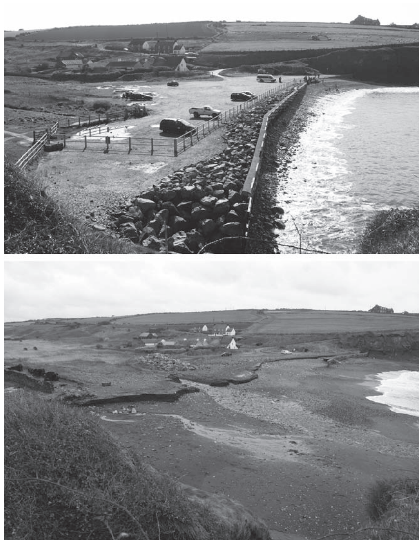
Figure 6.4. Aber-eiddi, Pembrokeshire – disappearing coast and workers' cottages. Top: the intact sea defence; Bottom: after the sea defence was breached by storms.
