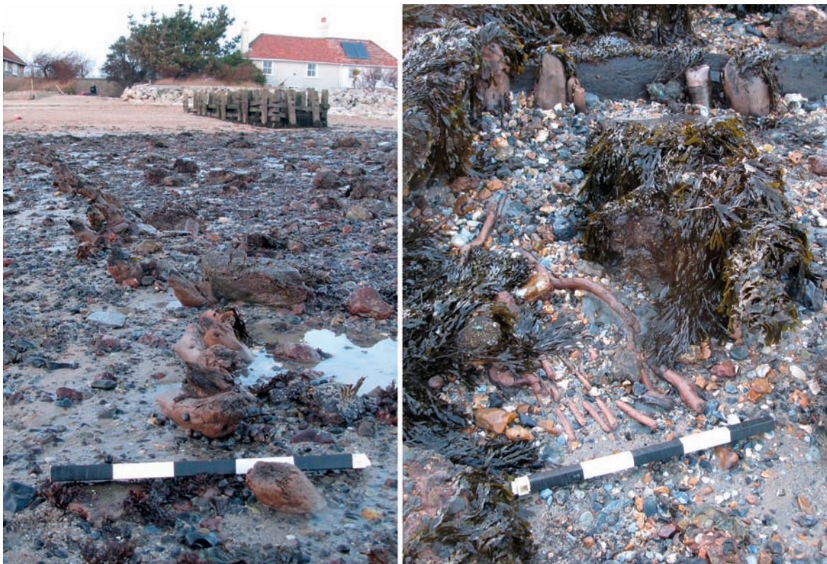
Figure 4.5. The old jetties at Pitts Deep, on the Solent, UK that were recorded in the 16th century are now degrading rapidly. Elements of timber structure are now clearly visible (left image) while storms in 2015 exposed new areas of wattle as the protective jetty infill deposits are being dispersed (right) (Photo: G. Momber, MAT).
