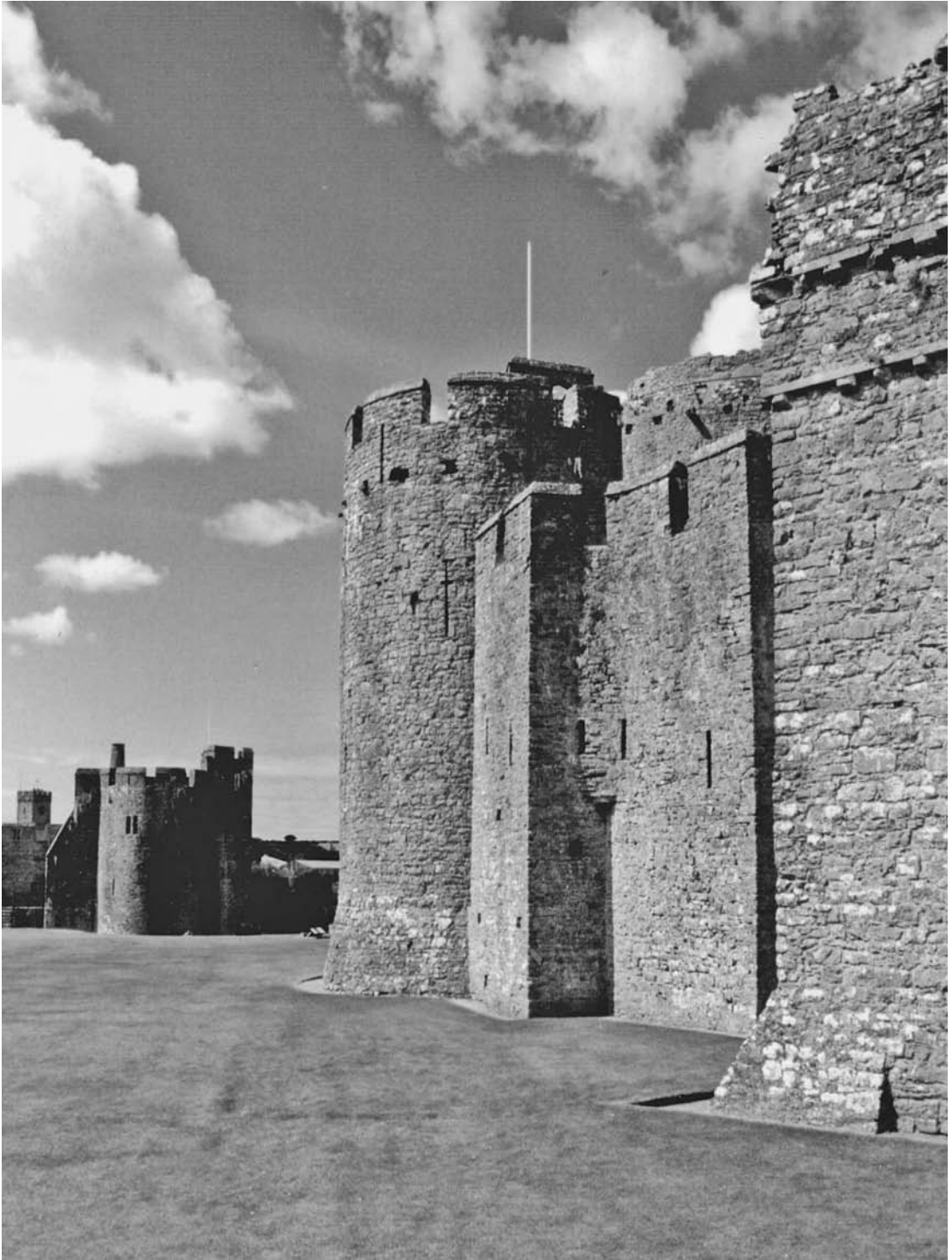
Round towers improved a castle's ability to withstand bombardment by catapulted missiles and undermining by enemy sappers. William de Valence added the round dungeon at Pembroke Castle in the late thirteenth century.
