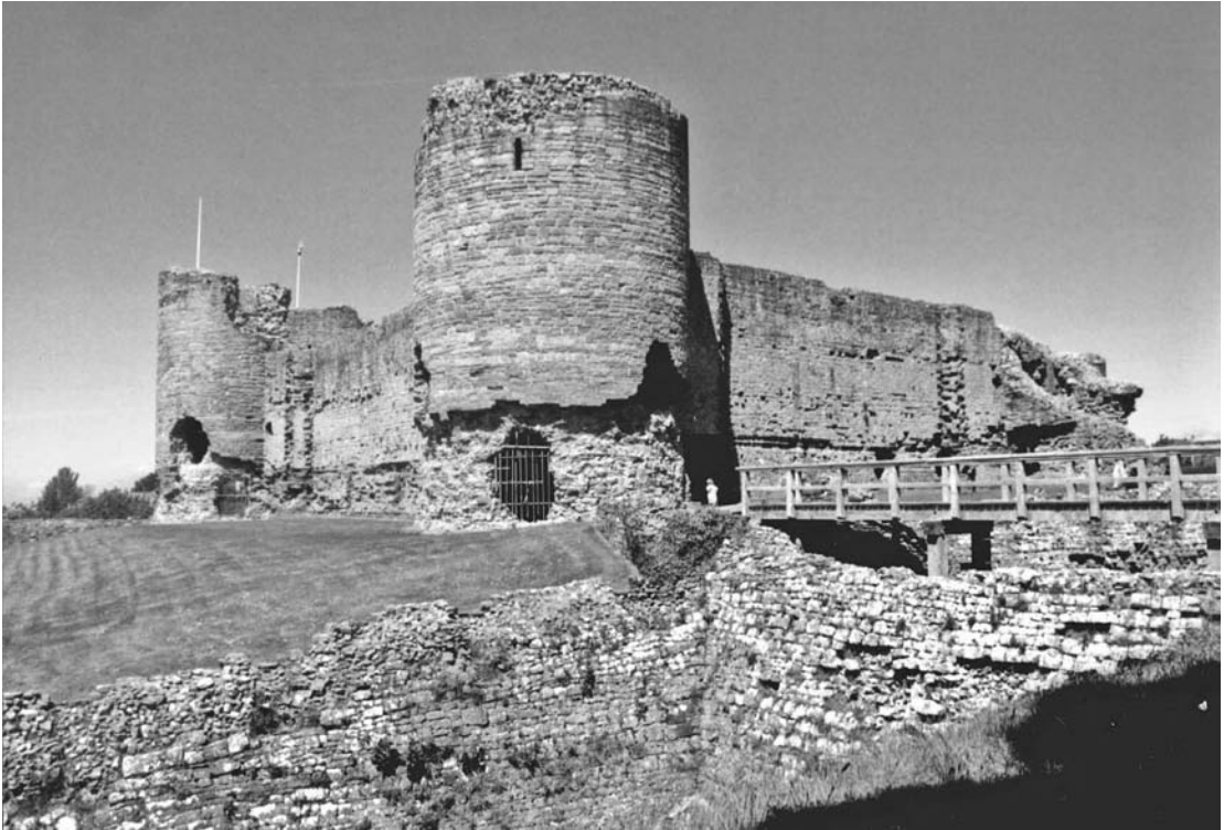
The great round towers at Rhuddlan Castle splendidly demonstrate the differences between ashlar and rubble building stone.
