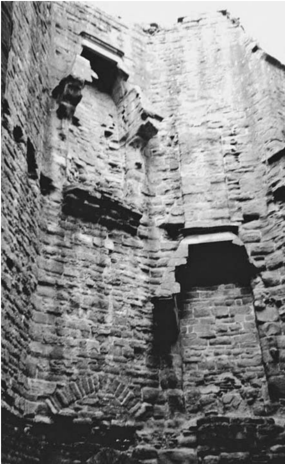
Even though a building may be an empty shell, the different stories can be distinguished by the placement of certain features, such as these fireplaces.
