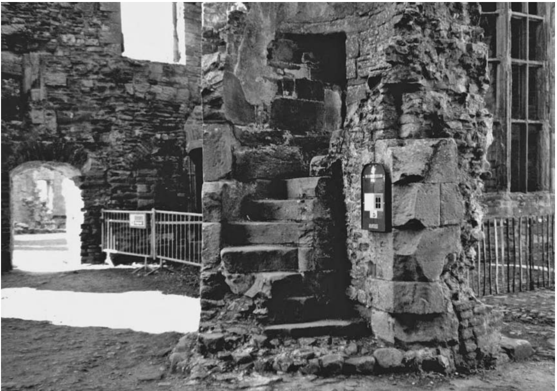
Originally leading into the first floor of the great hall from an antechamber, this spiral staircase at Raglan Castle now seems to lead to the heavens. Ashlar blocks and the rubble core are visible on the exterior.
