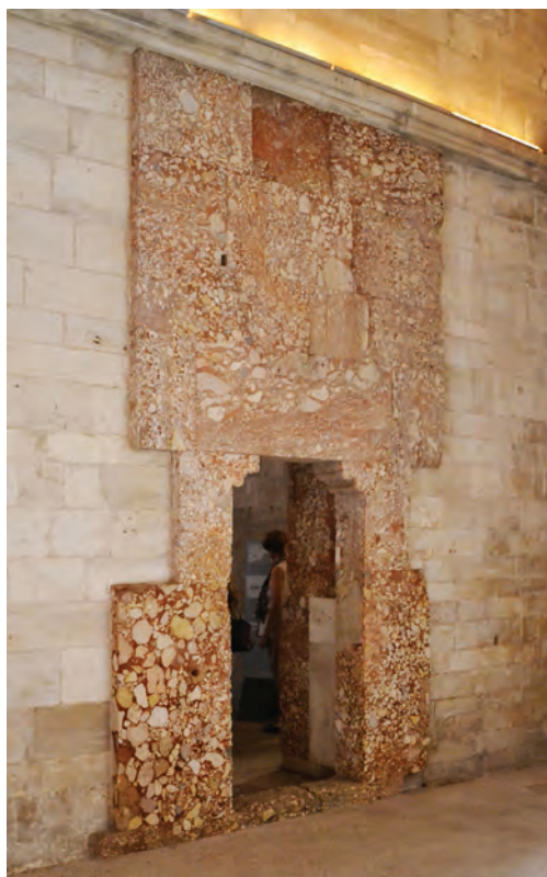
Fig. 10.4. Castel del Monte (Puglia) – A remnant of the red breccia with which the walls of the ground-floor rooms of the castle were faced (second quarter of the thirteenth century).
