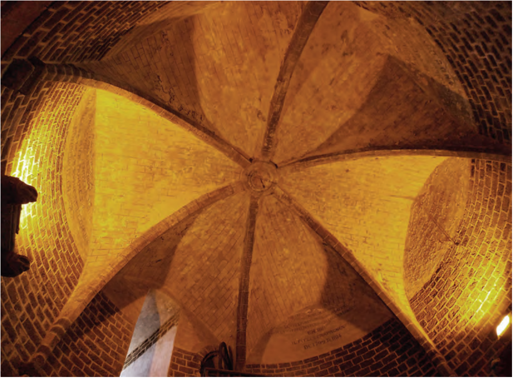
Fig. 4.20. Verneuil-sur-Avre (Haut-Normandie) Sexpartite ribbed vault over the ground storey of the great tower (first quarter of the thirteenth century).
