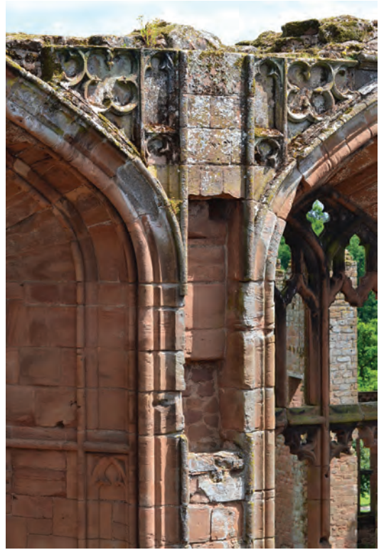
Fig. 3.12. Kenilworth (Warwickshire) Chase for securing one of the roof trusses in the great hall (third quarter of the fourteenth century).
