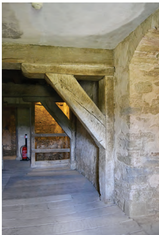
Fig. 3.3. Stokesay (Shropshire) Bracing system for the main beams over the ground floor of the solar block (last quarter of the thirteenth century).
