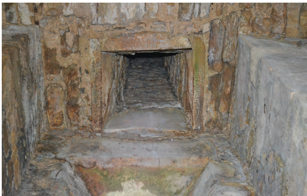
Fig. 9.8. Castle Bolton (Yorkshire) Flue in the head of a window in the ground-floor bakehouse (last quarter of the fourteenth century).
