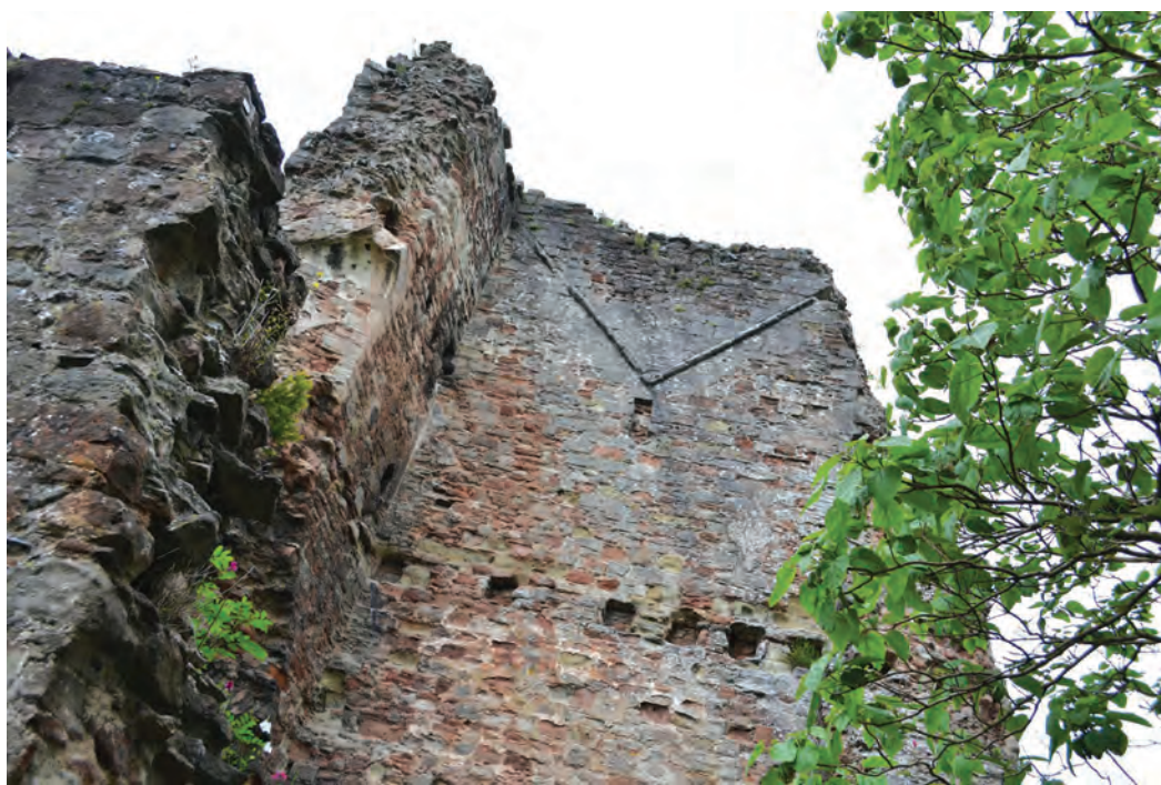
Fig. 3.4. Bridgnorth (Shropshire) The early twelfth century great tower has an unusual inverted roof profile. The technique was also used in the early keep of Portchester and may be a product of a regional school of carpentry.
