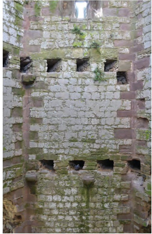
Fig. 3.7. Rhuddlan (Flintshire) The hexagonal interior of one of the corner towers, showing the alternating orientations of the beam sockets (fourth quarter of the thirteenth century).
