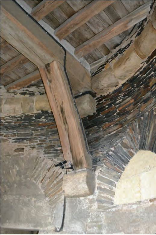
Fig. 3.6. Angers (Maine-et-Loire) The flooring arrangement of the Windmill Tower in which the joists rested on top of a pair of main beams, which were themselves strengthened by corbels and braces (second quarter of the thirteenth century).
