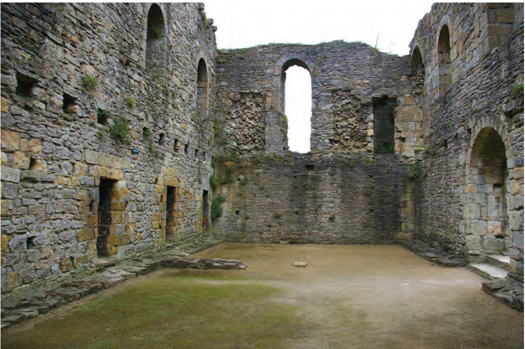
Fig. 3.2. Richmond (Yorkshire) Scolland's Hall from the east, showing the sockets for the first-floor main beam (in the centre of the end wall) and joists (in the two side walls) (third quarter of the eleventh century).
