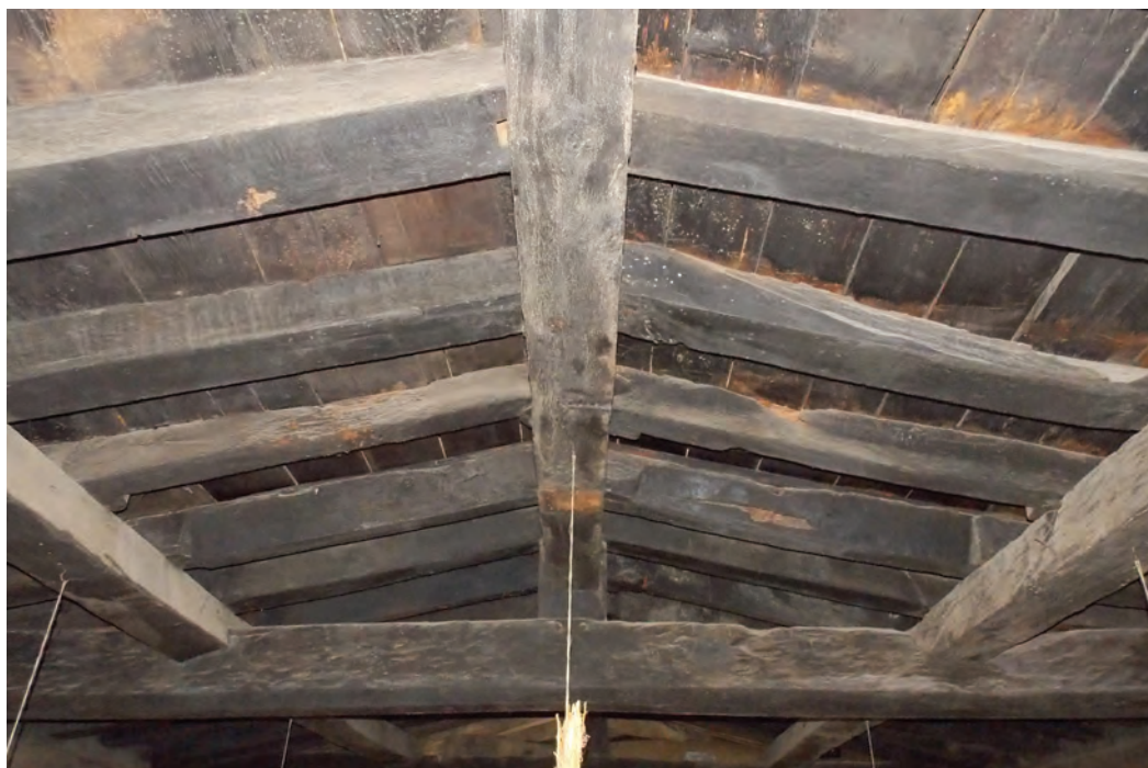
Fig. 3.13. Carlisle (Cumberland) Roof over the hall of the outer gatehouse made by the carpenter William Wright of Lancaster (c. 1381).
