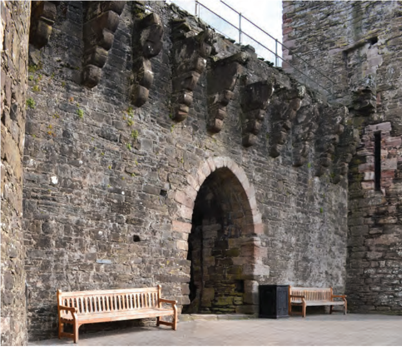
Fig. 7.17. Conwy (Caernarfonshire) Machicolations over the gateway to the outer ward (last quarter of the thirteenth century).
