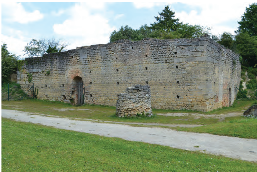
Fig. 5.1. Doué-la-Fontaine (Maine-et-Loire) The ground-floor hall which was later raised into a great tower and encased within a motte (second half of the ninth century).
