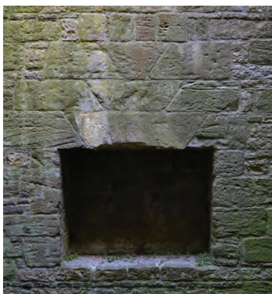
Fig. 4.14. Caernarfon (Gwynedd) Fireplace in the Well Tower with three tiers of joggling (last quarter of the thirteenth century).
