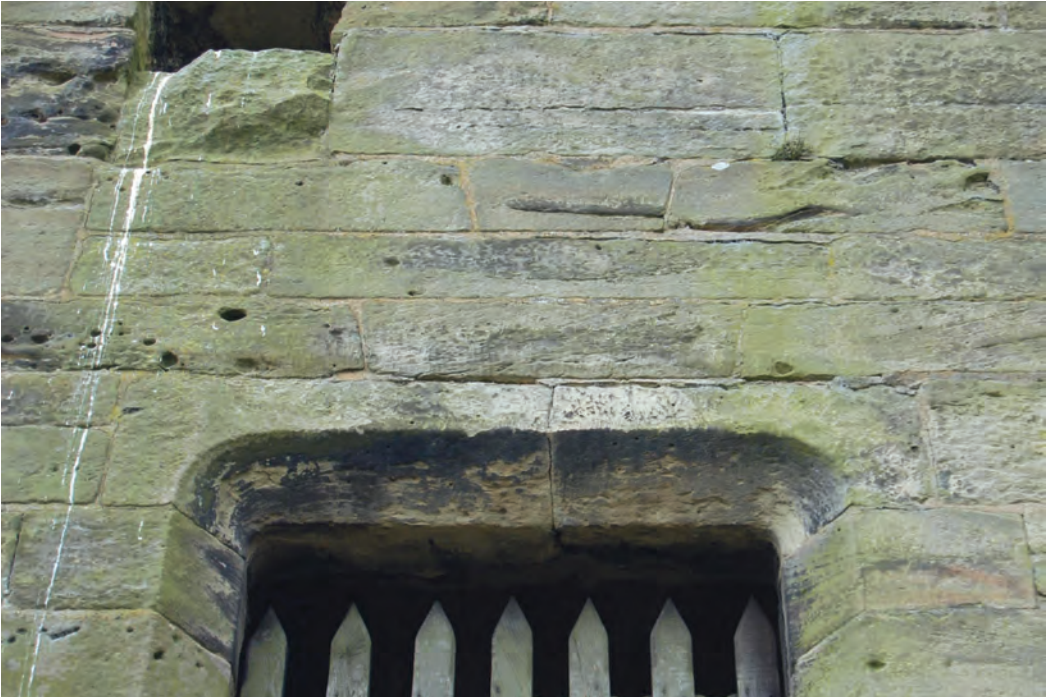
Fig. 4.15. Tutbury (Staffordshire) Successive wedge-shaped stones above a doorway in the North Tower designed to relieve pressure on the lintel ( c. 1441–1450).
