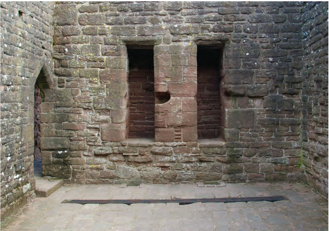
Fig. 8.13. Goodrich (Herefordshire) Twin windlass niches in the main gateway with holes for the portcullis chains in the floor beneath them and a slot for a second portcullis in the foreground (last quarter of the thirteenth century).
