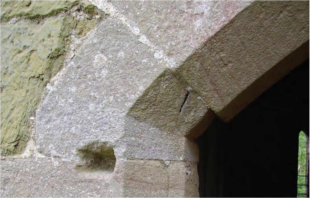
Fig. 4.9. Stokesay (Shropshire) Detail of the entrance to the great tower showing slippage between the springer and voussoir, and a crack in the springer (last decade of the thirteenth century).
