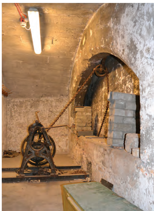
Fig. 8.12. Lancaster (Lancashire) Portcullis chamber in the main gatehouse (first quarter of the fifteenth century with nineteenth-century winch).
