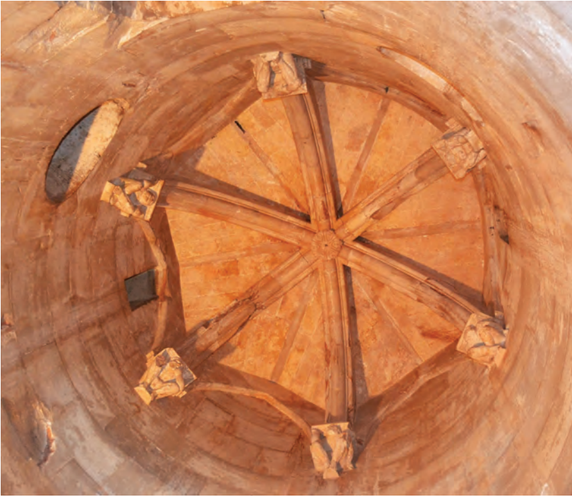
Fig. 4.25. Castel del Monte (Puglia) Sexpartite vault over a stairwell (second quarter of the thirteenth century).
