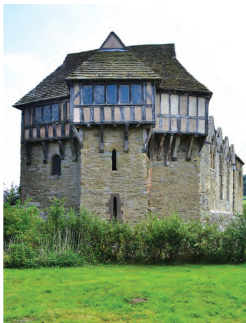
Fig. 3.16. Stokesay (Shropshire) Oversailing timber upper storey around the north tower (c. 1290).
