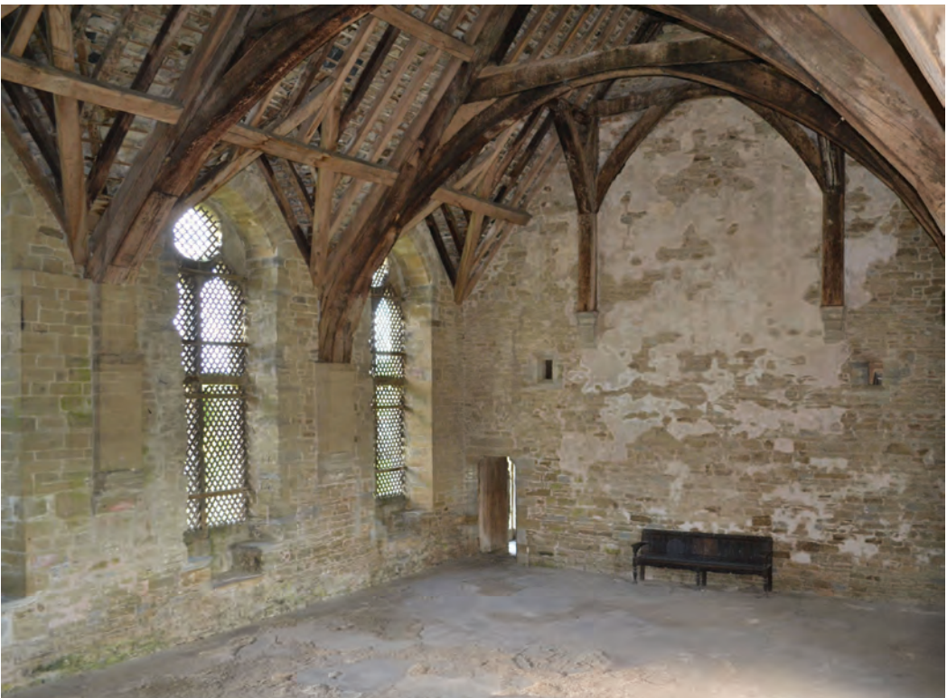
Fig. 3.10. Stokesay (Shropshire) The great hall from the north west with an end truss of aisled construction and main trusses of cruck construction. The feet of the crucks have been truncated and the stone corbels on which they rest extended upward to compensate; originally the crucks would have extended most of the way down the walls ( c. 1280).
