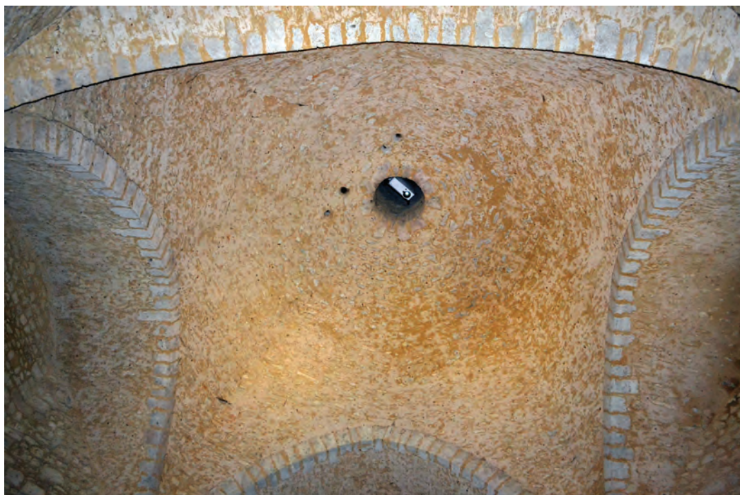
Fig. 4.18. Provins (Seine-et-Marne) – Domed sail vault over the first floor of the Tour de César (third quarter of the twelfth century).
