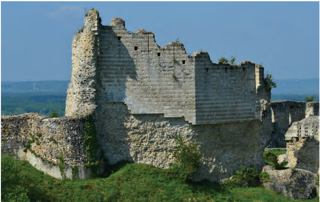
Fig. 10.1. Château Gaillard (Eure) - The curtain around the outer ward of was decorated with alternating courses of red and white masonry (1196–1198).
