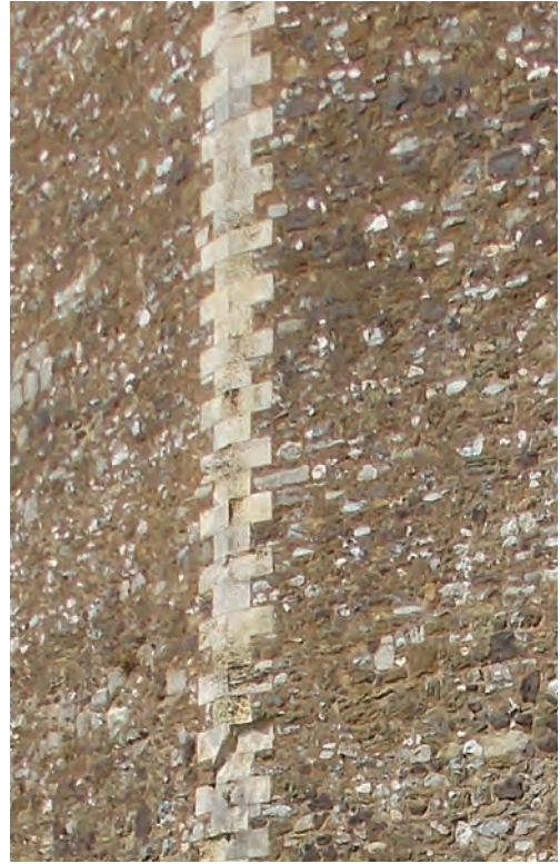
Fig. 4.7. Dover (Kent) Stitching at an angle of the inner curtain wall at Dover (c. 1168–1189).
