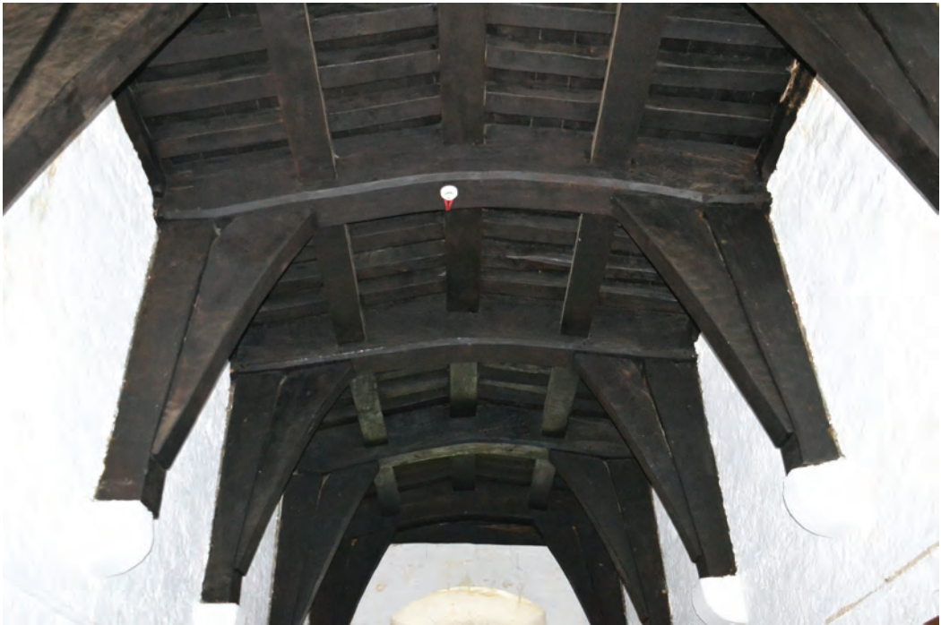
Fig. 3.14. Lancaster (Lancashire) Roof over the gatehouse (first quarter of the fifteenth century).
