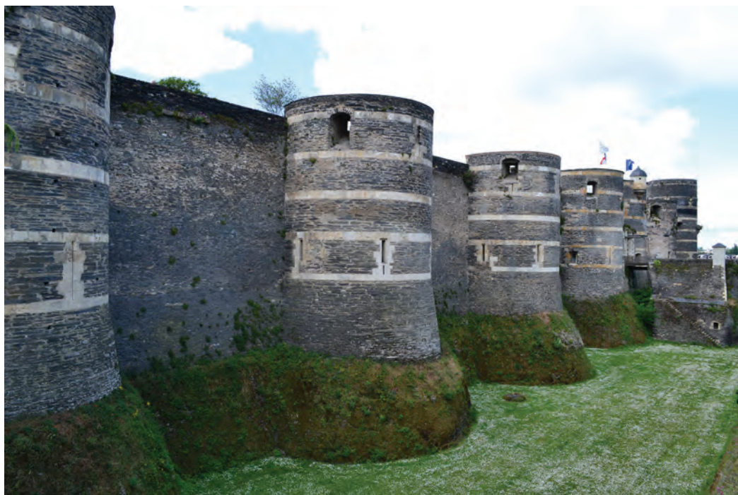
Fig. 10.2. Angers (Maine-et-Loire) The builders of the castle created a striking contrast by interspersing the local black schist rubble with bands of limestone ashlar.
