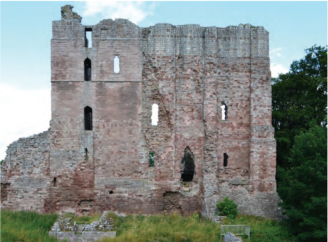
Fig. 5.10. Norham (Northumberland) The south-east elevation of the great tower attributed to Richard Wolveston. The greater part of the stonework in this elevation dates from the third quarter of the twelfth century, but the tower has been subjected to fifteenth century rebuilding (left) and heightening.
