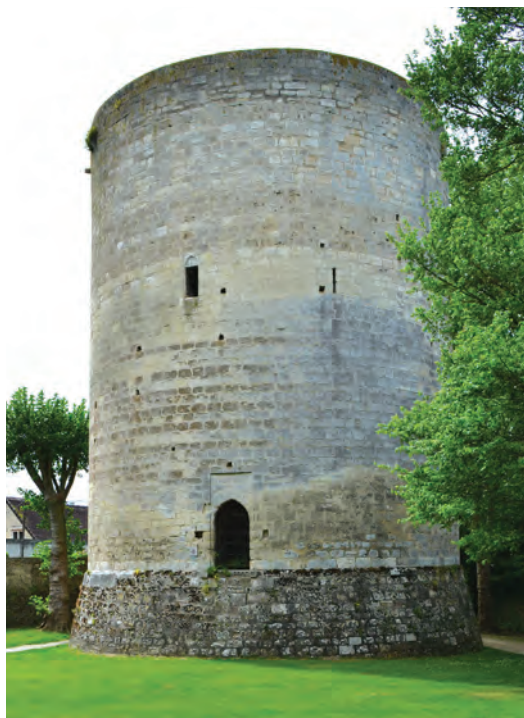
Fig. 4.5. Villeneuve-sur-Yonne (Yonne) One of several tours philippiennes in which the builders employed scaffolding in a spiral pattern around the tower, the evidence for which are the two lines of putlog holes ascending from left to right in an anti-clockwise direction (1205–1212).
