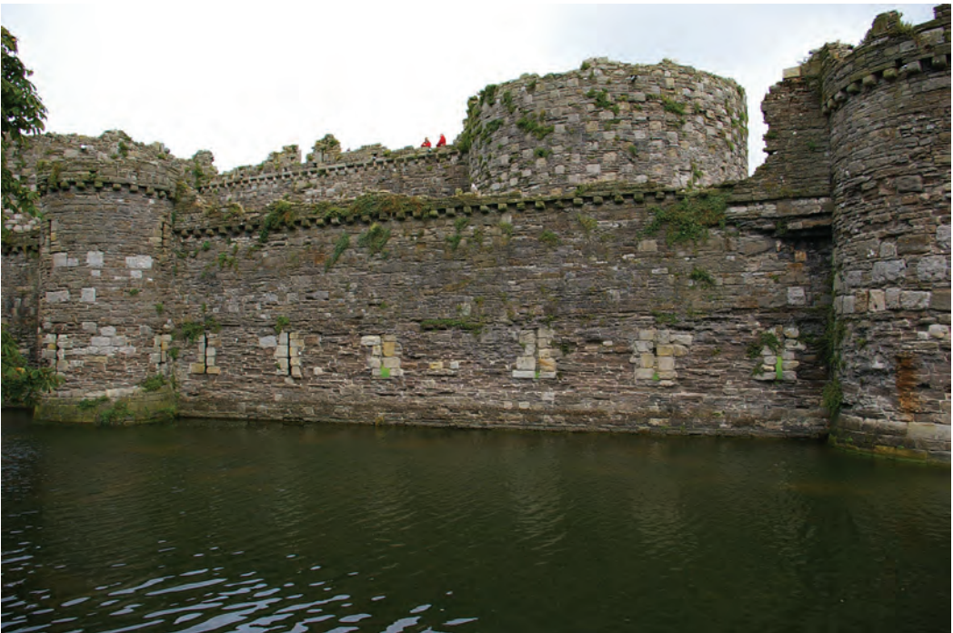
Fig. 7.14. Beaumaris (Anglesey) The line of arrow loops along the west curtain with the defences of the inner ward looming up behind.
