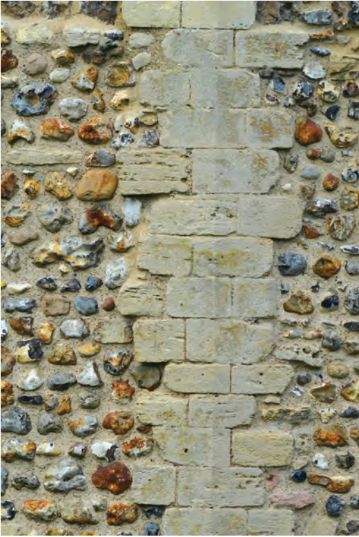
Fig. 4.6. Framlingham (Suffolk) Stitching at the junction of two sections of curtain wall (last decade of the twelfth century).
