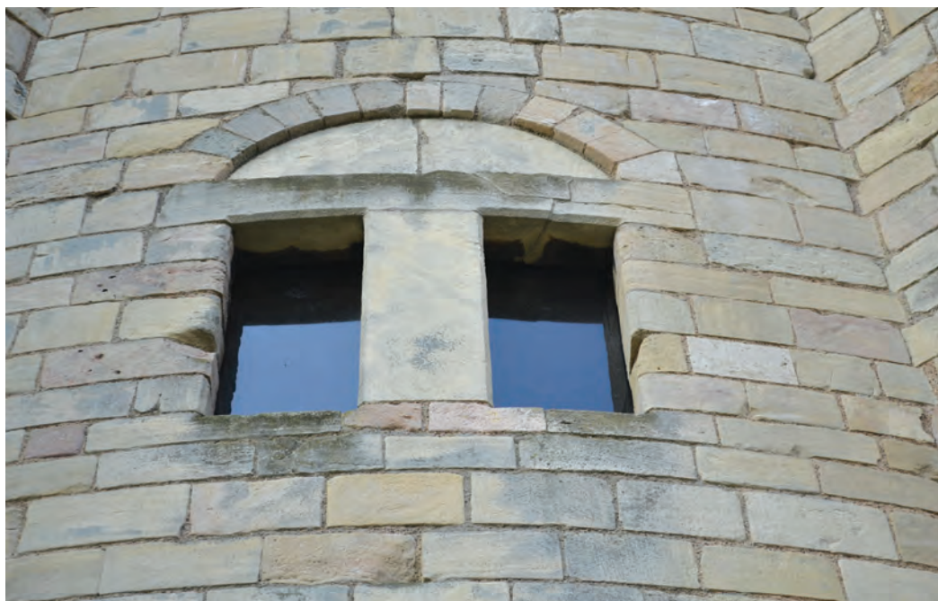
Fig. 4.17. Conisbrough (Yorkshire) Window in the keep with broad mullion, common lintel, split tympanum and relieving arch. Note that the lintel has failed and has had to be repaired (last quarter of the twelfth century).
