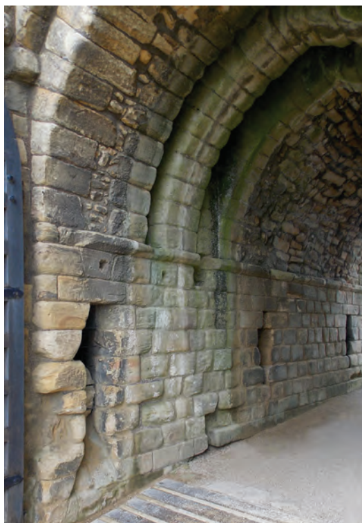
Fig. 8.14. Warkworth (Northumberland) The portcullis slot of the main gateway extends only to the top of the string course. Behind it is a machicolation slot.
