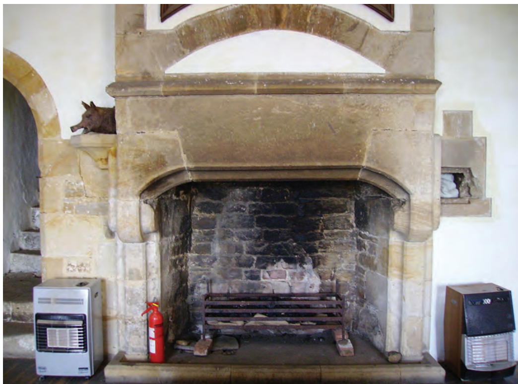
Fig. 4.13. Castle Bolton (Yorkshire) Fireplace in the south-west tower with joggled lintel on corbelled haunches (last quarter of the fourteenth century).
