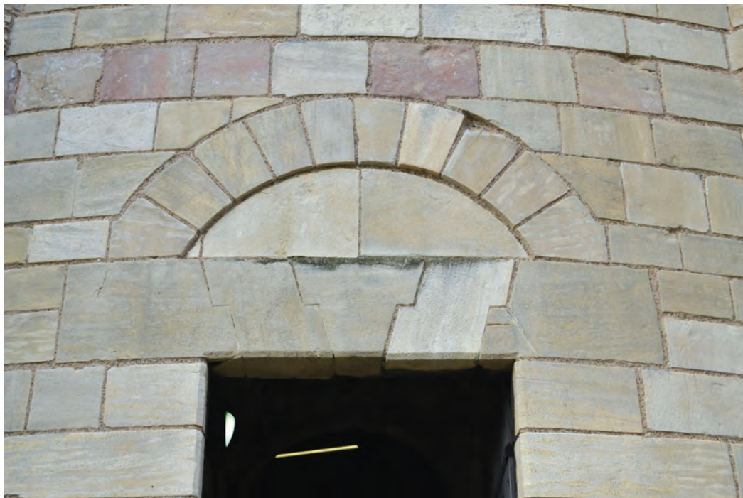
Fig. 4.11. Conisbrough (Yorkshire) Joggled lintel over the main entrance to the keep with split tympanum and relieving arch (last quarter of the twelfth century).
