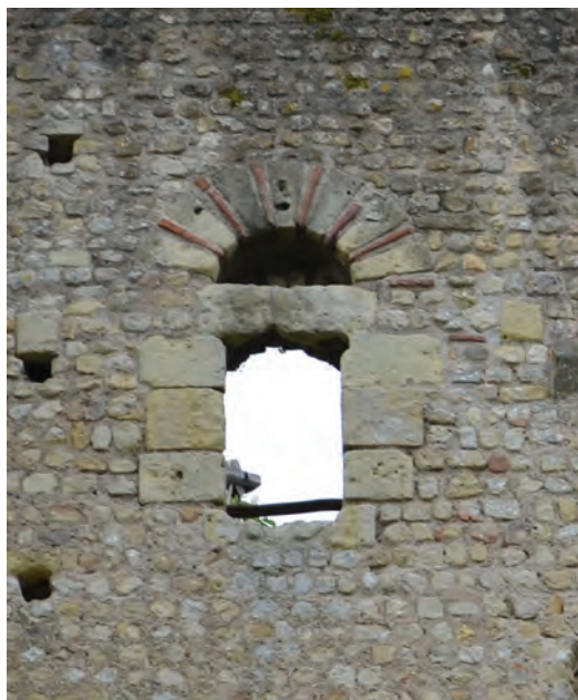
Fig. 4.16. Langeais (Indre-et-Loire) Lintelled window with relieving arch in the great tower ( c. 1000).
