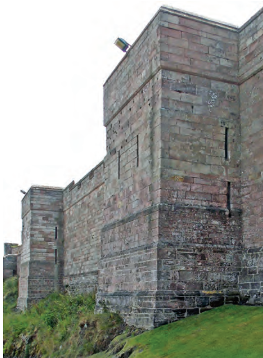
Fig. 7.3. Bamburgh (Northumberland) The wall towers of the inner ward from the north west, perhaps by the mason, Maurice (third quarter of the twelfth century).
