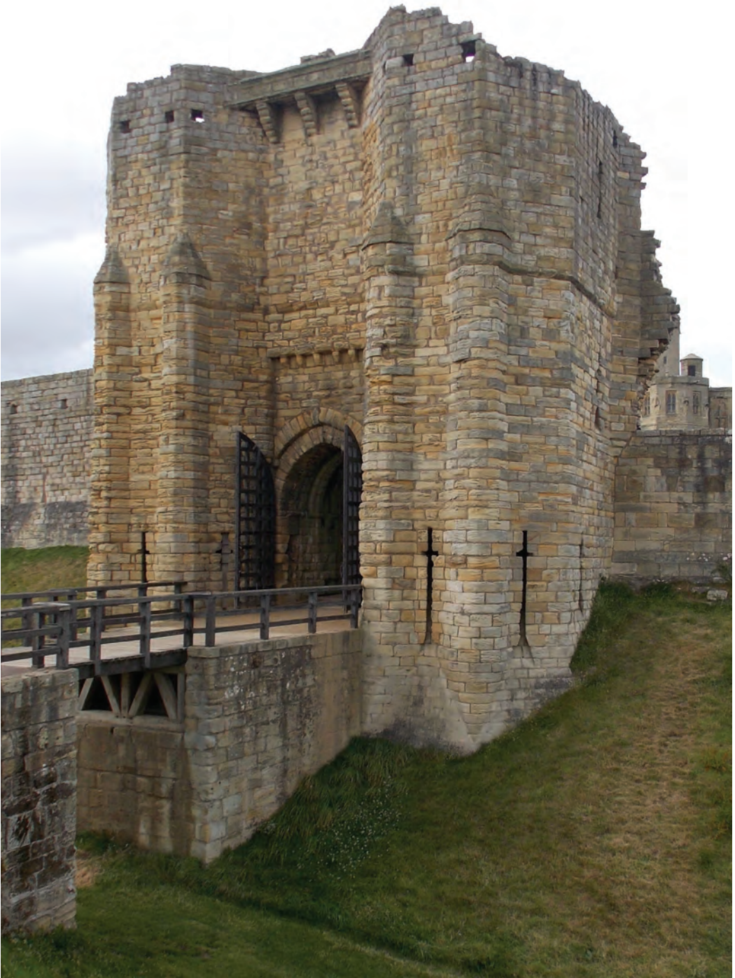
Fig. 10.14. Warkworth (Northumberland) The gatehouse of c. 1200 from the south east; the uppermost storey is an addition of c. 1400.
