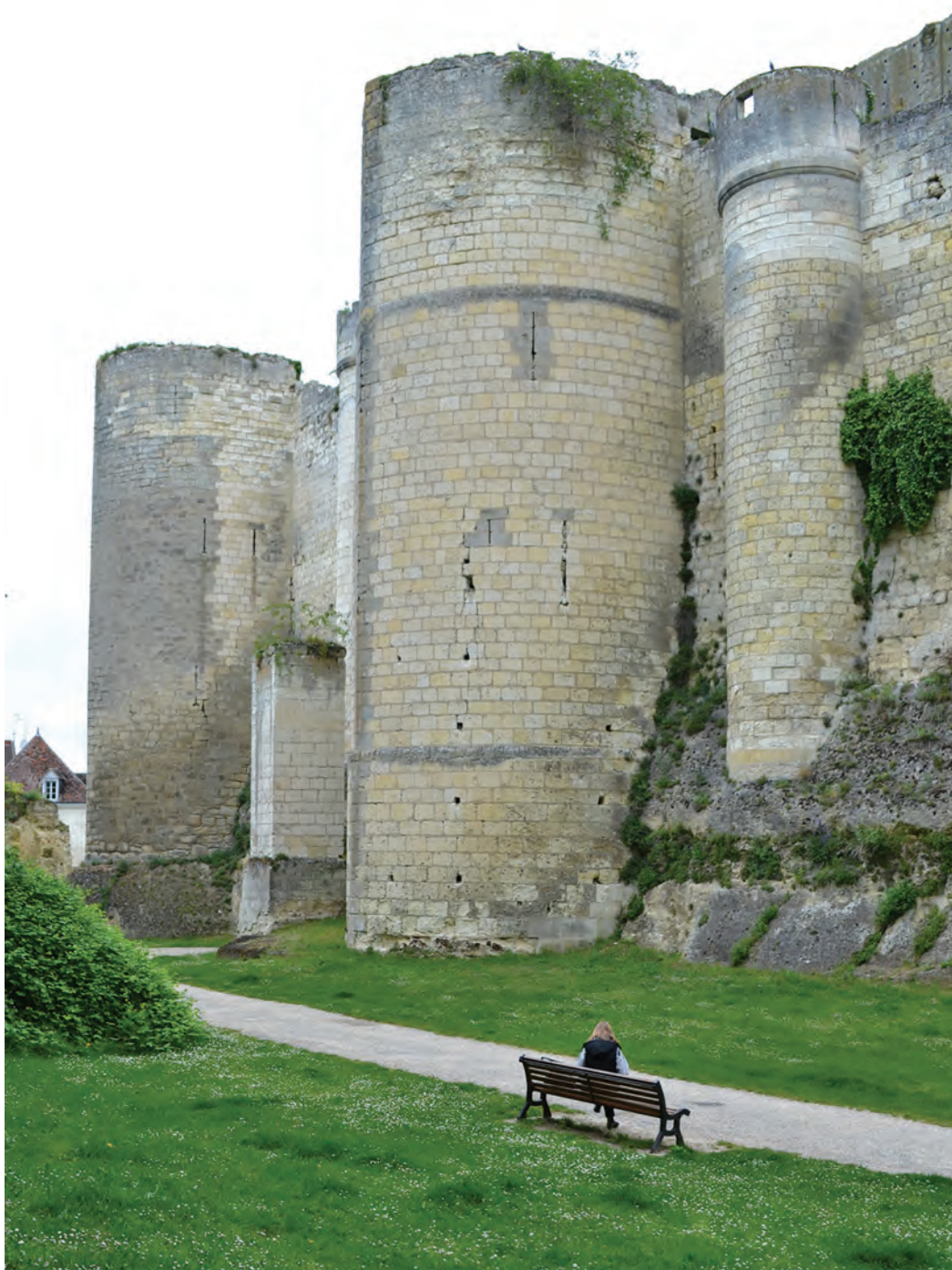
Fig. 7.10. Loches (Indre-et-Loire) A semi-circular turret of Henry II (last quarter of the twelfth century) in juxtaposition with later beaked towers (last decade of the twelfth century or first decade of the thirteenth century).
