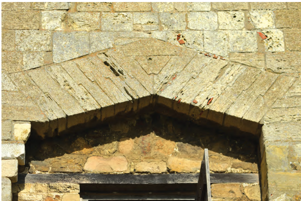
Fig. 4.10. Orford (Suffolk) Joggled gate arch to the great tower (third quarter of the twelfth century).
