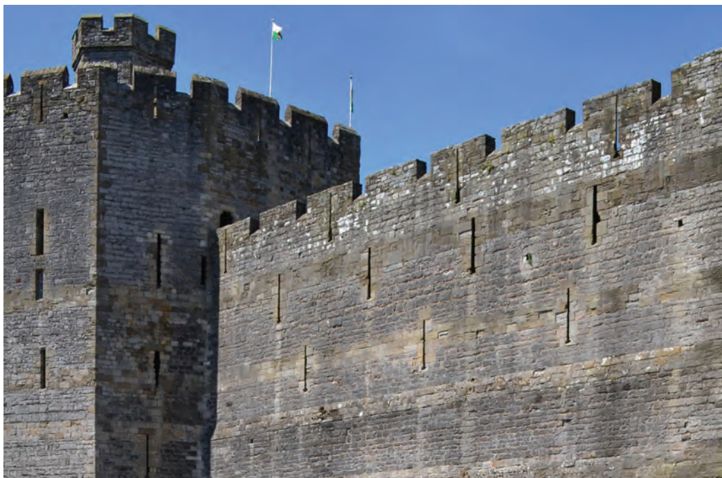
Fig. 7.15. Caernarfon (Caernarvonshire) Three tiers of arrow loops manned from the parapet and two intra-mural galleries.
