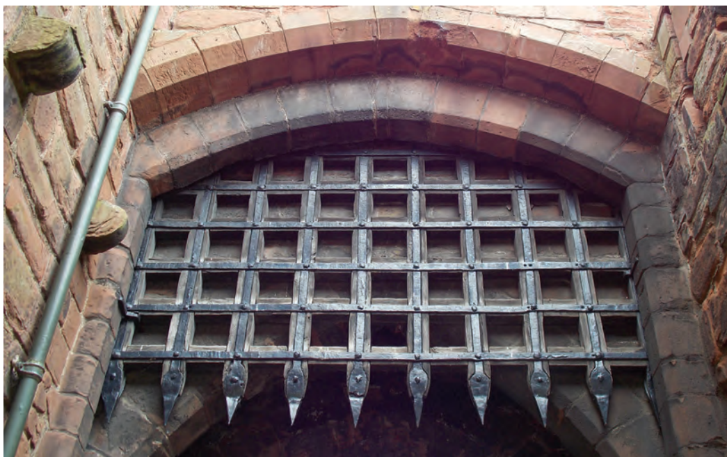
Fig. 8.11. Carlisle (Cumberland) The iron clad portcullis (1378–1383).
