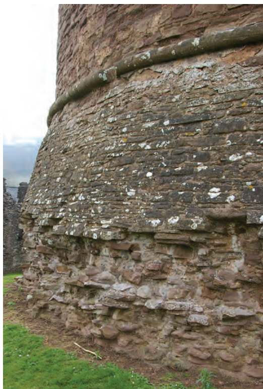
Fig. 4.1. Skenfrith (Monmouthshire) Battered plinth of the great tower with bold roll moulding at first-floor level (first third of the thirteenth century).
