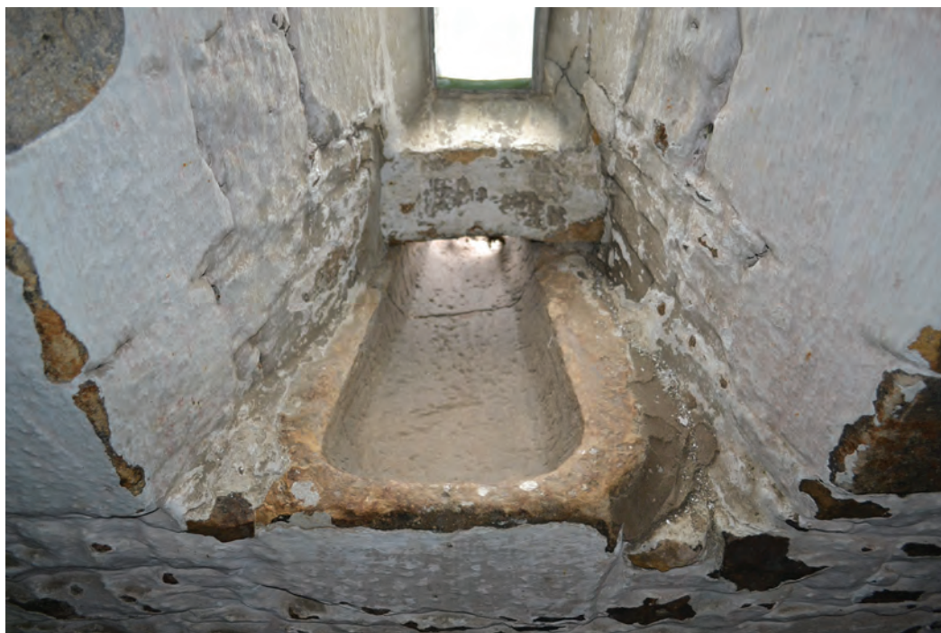
Fig. 9.13. Castle Bolton (Yorkshire) Sink/urinal draining to an external spout (last quarter of the fourteenth century).
