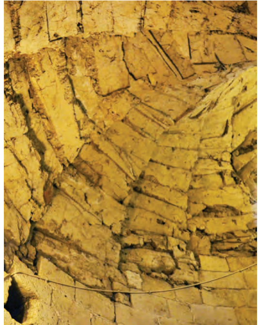
Fig. 4.23. Orford (Suffolk) – Plank marks of the formwork on the stair vault (third quarter of the twelfth century).
