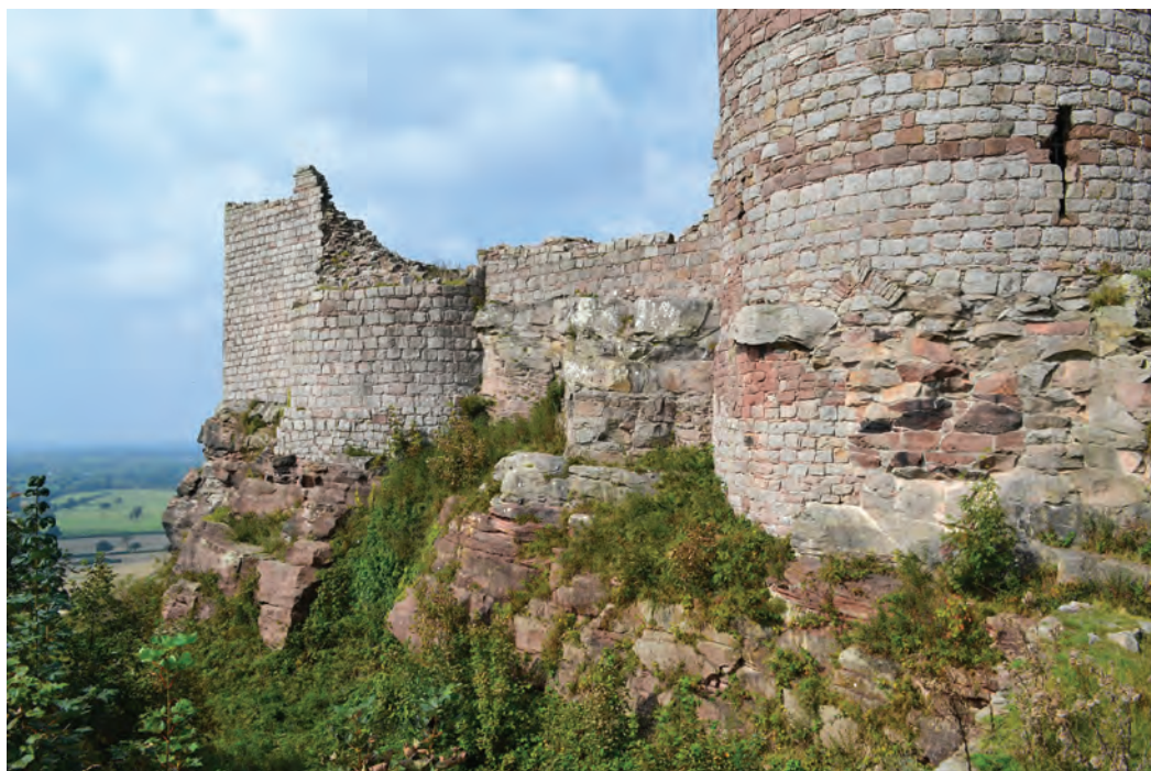
Fig. 2.2. Beeston (Cheshire) The inner ward enceinte perched on the edge of the rock-cut ditch from the north ( c. 1220).
