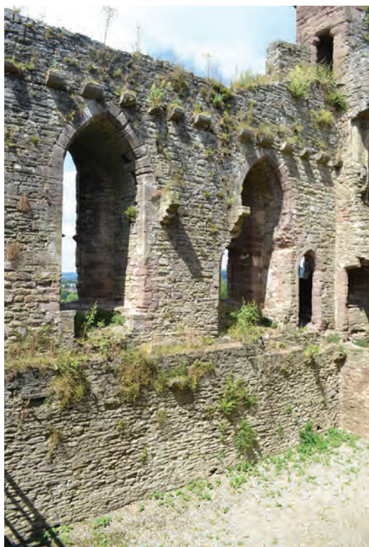
Fig. 3.11. Ludlow (Shropshire) The late thirteenth-century great hall showing two tiers of corbels; the lower ones carried the bracing for the main roof trusses, and the upper ones wall plates into which the feet of the rafters would have been jointed (last quarter of the thirteenth century).
