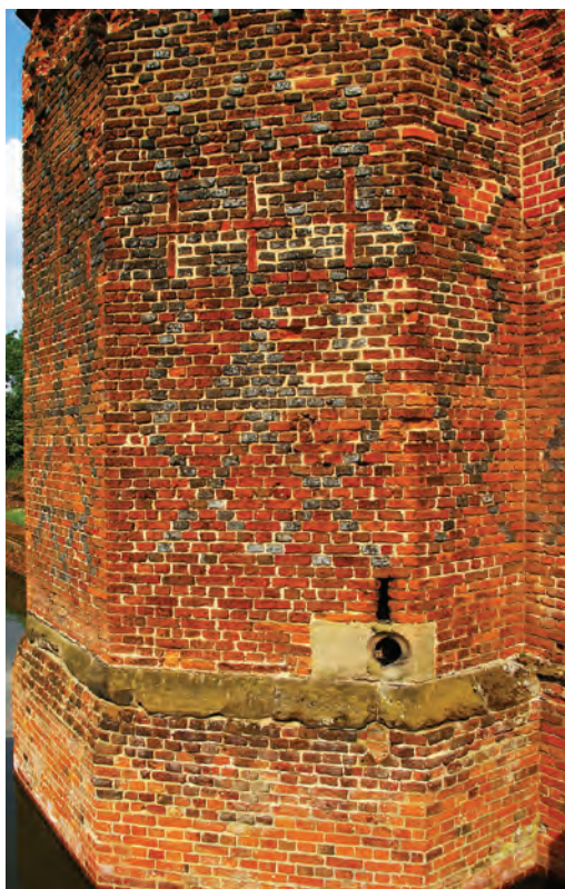
Fig. 10.5. Kirby Muxloe (Leicestershire) Patterning made by bricks of contrasting colours on one of the gatehouse towers (1481–1483).
