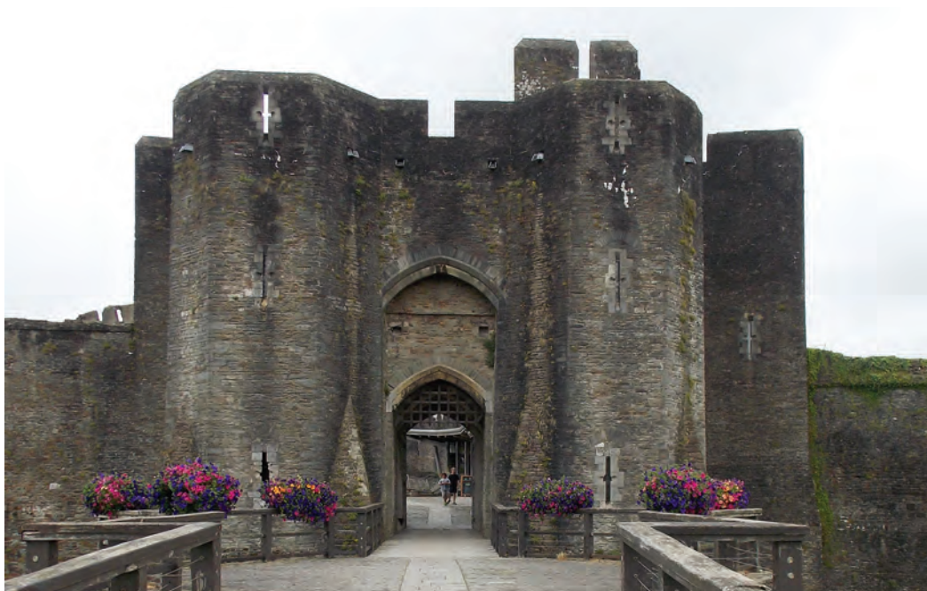
Fig. 8.9. Caerphilly (Glamorganshire) The main outer gateway with holes for the drawbridge chains above the gateway (last quarter of the thirteenth century).
