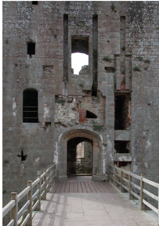
Fig. 8.10. Raglan (Monmouthshire) Amidst later alterations, the entrance to the keep retains the slots for the counterbalance beams that were used in operating two drawbridges. The system allowed pedestrian access while keeping the main gateway closed.
