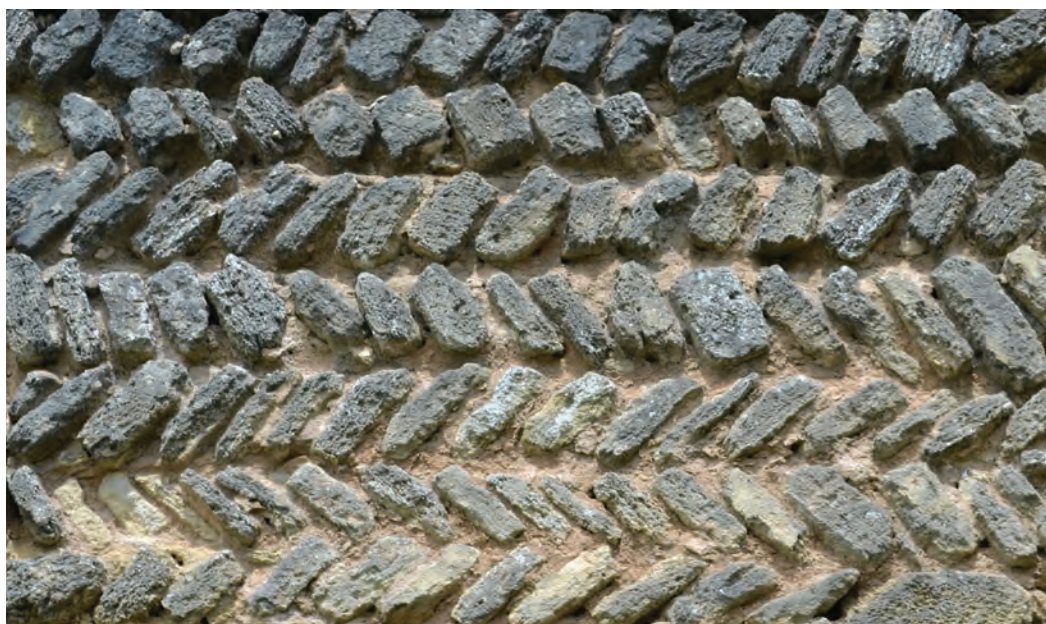
Fig. 4.3. Doué-la-Fontaine (Maine-et-Loire) Herringbone masonry (last quarter of the ninth century).
