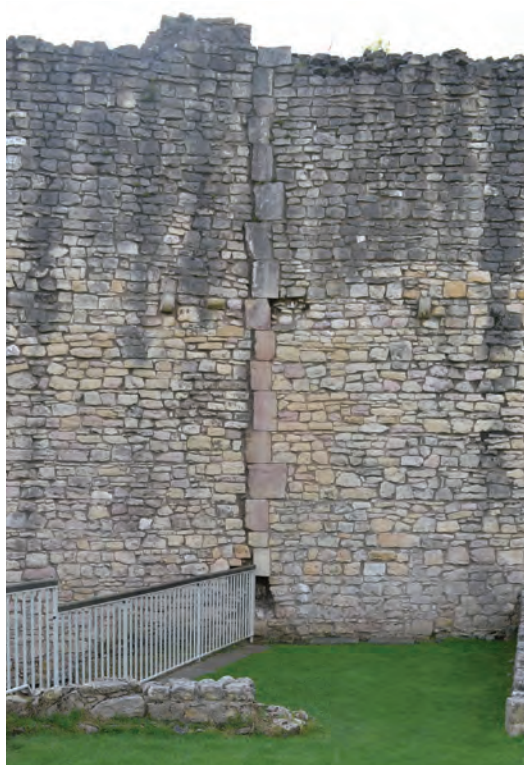
Fig. 4.8. Conisbrough (Yorkshire) Stitching between two sections of curtain wall (last decade of the twelfth century).
