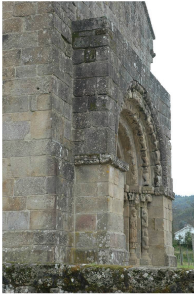
Figure 8.6 Church of the Saviour of Bravães, stonemasonry structure thickening the western façade.
