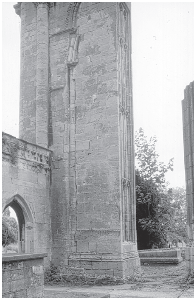
FIG. 7. Croyland Abbey: east end of south nave arcade, showing inserted 13th-century respond
