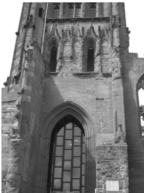
FIG. 10. Coventry, St Michael's: west tower, east elevation showing primary and secondary roof lines
