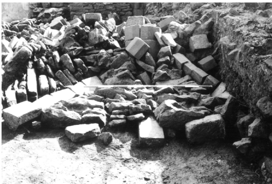
FIG. 5. St Mary's Cathedral Priory: the tumbled vaults of the refectory undercroft. An octagonal pier is visible in the centre: scale 2m
