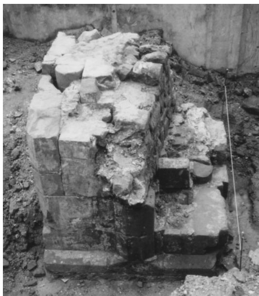
FIG. 5. Coventry, Cathedral Church: north transept pier, from the south, with the masonry reinforcement added in the 14th century
