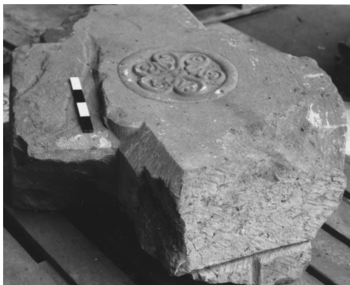
FIG. 15. Coventry, Cathedral Church: the key-stone for a vault with square-section ribs (scale 20cm) Photo, R. K. Morris
