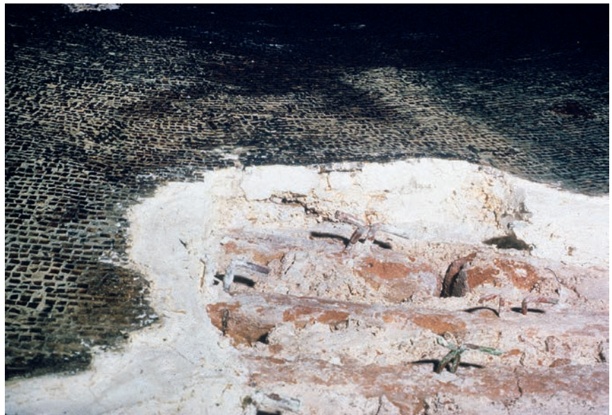
Figure 22 Detail of masonry, clamps and plaster layers with mosaic from the apse of Hagia Sophia, Istanbul, ninth century.
