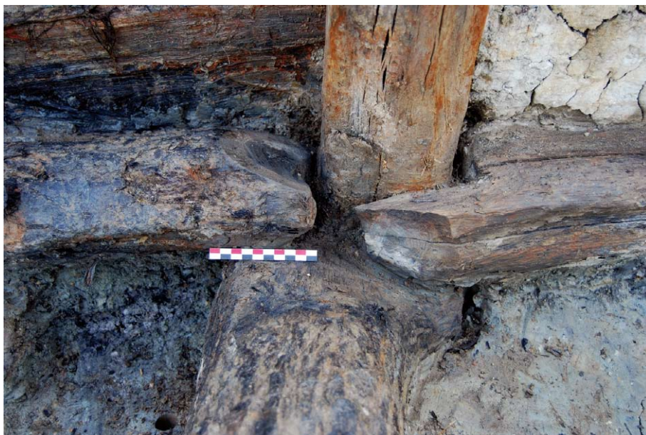
Fig. 9.3. The joints in the timber-lined shafts of Iron Age date at Băile Figa, Beclean, Romania (photo: Author)
