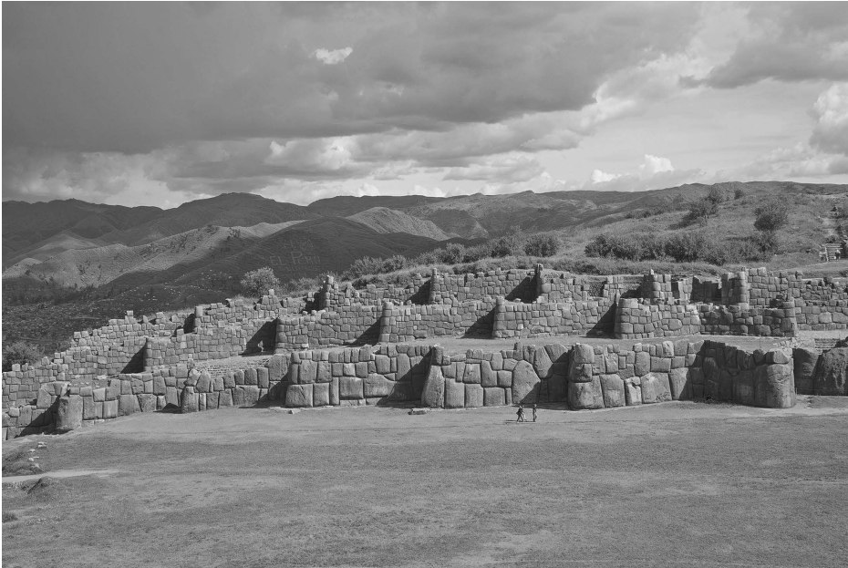
Figure 14.14 The Sacsahuaman fortress near Cuzco. Inca architecture was based on closely fitted stone blocks. They were moved by human hands since Andean llamas could only carry loads of about 45 kilograms (100 pounds). (Micajah/Thinkstock)
