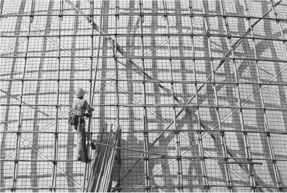
Figure 3.7 Bamboo scaffolding in use to build a modern high-rise. Asians have used this flexible and versatile material since the earliest times.
