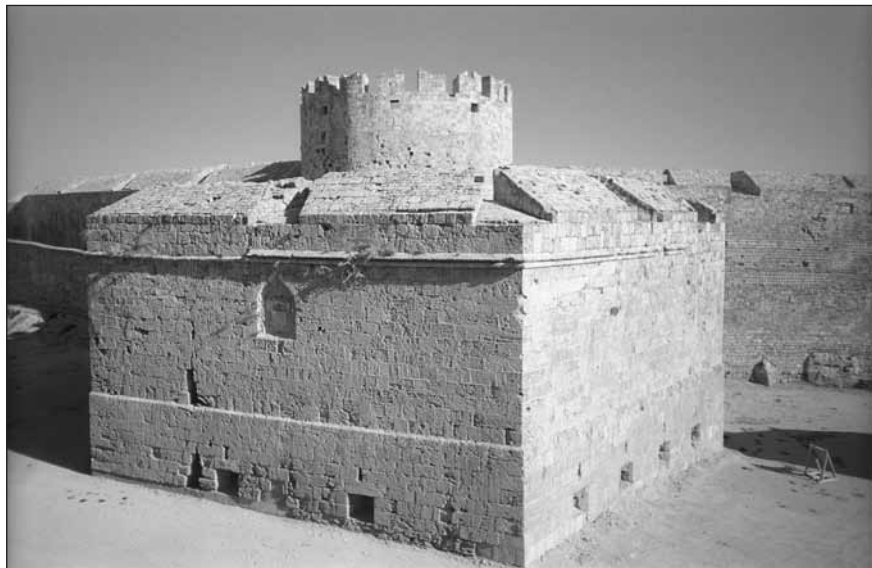
Figure 2.4 The tower of St. George, Rhodes. Built by master Fluvian (ca. 1421–1437) originally as part of a gate. Angled walls shielded the gate opening by 1465; after 1480, Masters d'Aubusson and Philippe Villiers de l'Isle Adam closed off the gate with thicker, bastion-like walls (Gabriel, Cité , 1:35–36). The tower demonstrates how the master and the convent continually updated the walls to meet the demands of improved gunpowder artillery. (Photo: Theresa Vann)
