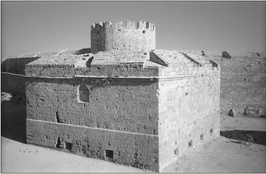
Figure 2.4 The tower of St. George, Rhodes. Built by master Fluvian (ca. 1421–1437) originally as part of a gate. Angled walls shielded the gate opening by 1465; after 1480, Masters d'Aubusson and Philippe Villiers de l'Isle Adam closed off the gate with thicker, bastion-like walls (Gabriel, Cité , 1:35–36). The tower demonstrates how the master and the convent continually updated the walls to meet the demands of improved gunpowder artillery. (Photo: Theresa Vann)
