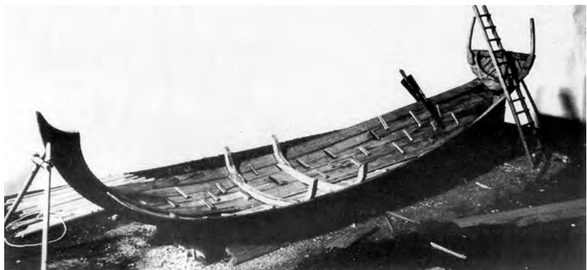
FIGURE 3.6. The bilges are now planked, guided by the bilge futtocks. At this stage, where the planks do not lie in one line next to each other, as in the previous stage, the planking tongs can only be used together with wedge-shaped filling chocks, filling the open space between planks and tongs. It is quite difficult to build a symmetrical hull shape with this technique. (Courtesy A. J. Hoving)
