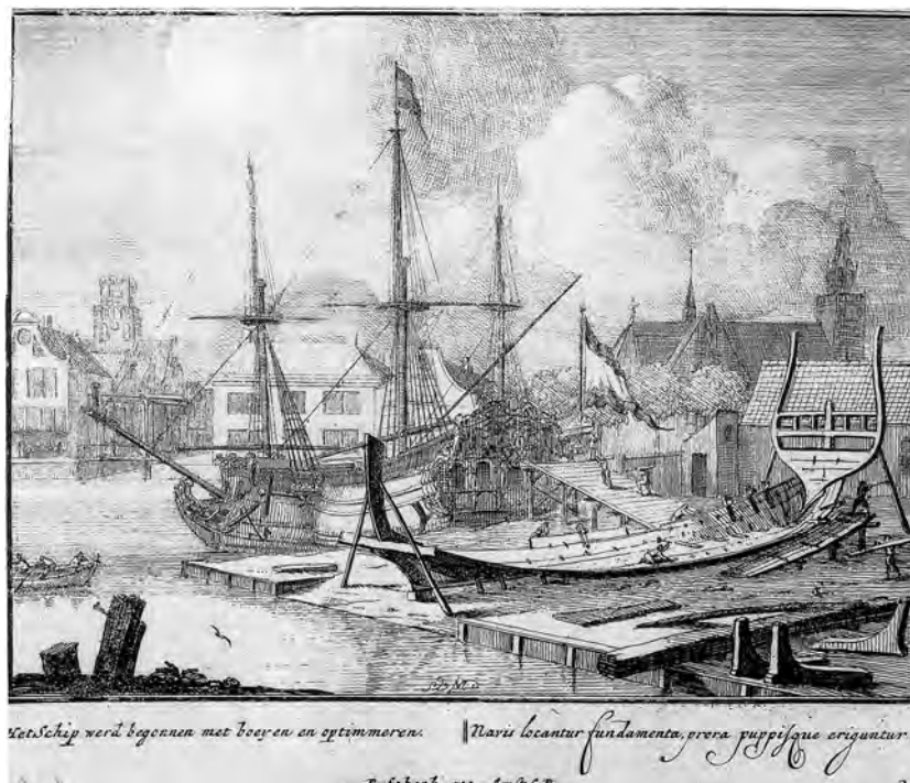
FIGURE 2.43. Siewert van der Meulen's late seventeenth-century engraving of the bottom of a ship on the stocks. The planking tongs are clearly visible.
