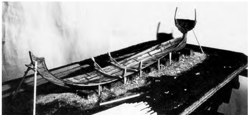
FIGURE 3.5. A floor timber and two bilge futtocks are raised at the location of the main frame. Because I was reluctant to believe Witsen at this stage, I even placed two floor timbers, although one would have sufficed. (Courtesy A. J. Hoving)
