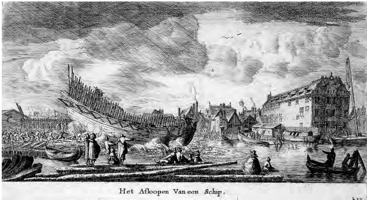
FIGURE 2.112. Etching of a ship launch by Reinier Nooms, 1660. The artist's depiction fits Witsen's description in all respects except one: the scaffolding supports are already attached. See section 59 (When it has been launched, then make scaffolding outside and to the stern). Courtesy Rijksmuseum, Amsterdam.
