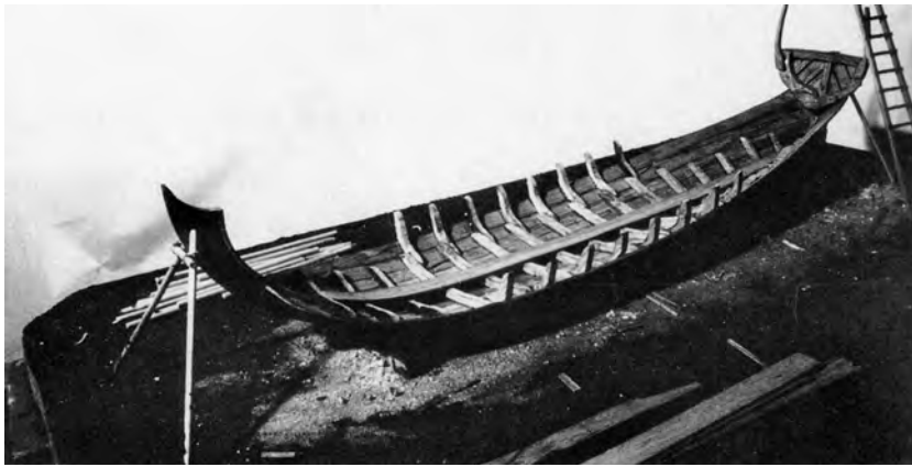
FIGURE 3.7. The shell formed by the bottom and the turn of the bilges is now filled with timbers. With a small vessel like this pleasure yacht, the frames do not lie close to each other as they do in larger vessels, but with wider spaces, as in launches and barges. (Courtesy A. J. Hoving)
