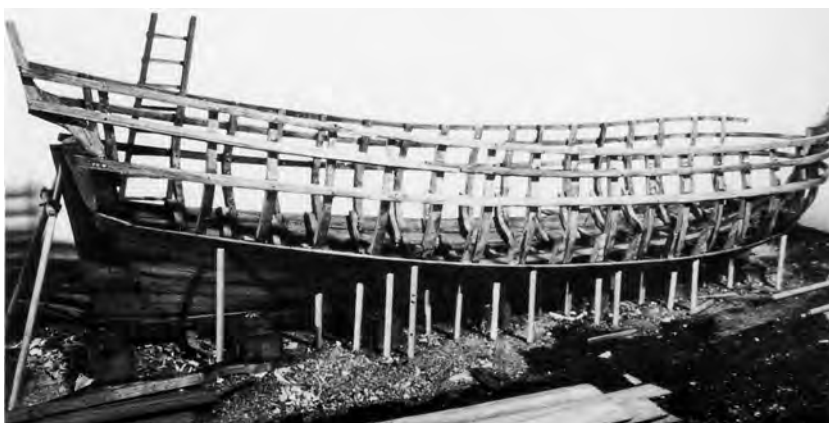
FIGURE 3.10. The other futtocks and top timbers are added. Above the master ribbands, other ribbands were used—first, to find the right shape of the frame timbers and, second, to keep them in place as the building process continued. The frame timbers were not joined together in any other way. (Courtesy A. J. Hoving)
