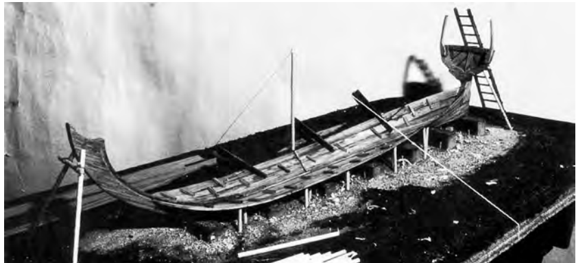
FIGURE 3.4. The bottom planking is continued with the aid of planking tongs. Wooden chocks keep the planks in place after they have been pressed edge to edge with the hook and chain (see “Tools” in chapter 1). Small wooden poles (shores) support the construction. (Courtesy A. J. Hoving)
