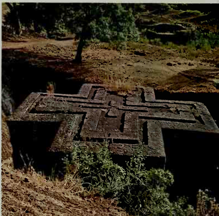
CONCENTRIC CROSSES are carved into the church's roof, which is almost exactly level with the surface of the ground from which the pit around it was excavated.
