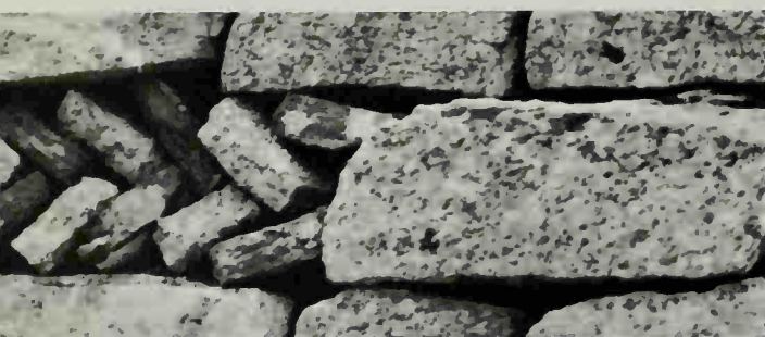
THREE DECORATIVE WALLS, built entirely without mortar, reflect the high level of construction that flourished in what is now Rhodesia. The chevron design at the top is from the ruins at Zimbabwe. The checkered and herringbone patterns below, probably the ruins of a chief's dwelling, were found at Naletale.
