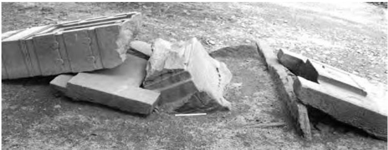
Fig. 52 The fallen remains of Stela 4 at Aksum, showing how the stela had originally been set in a socket lined with vertical slabs of stone
