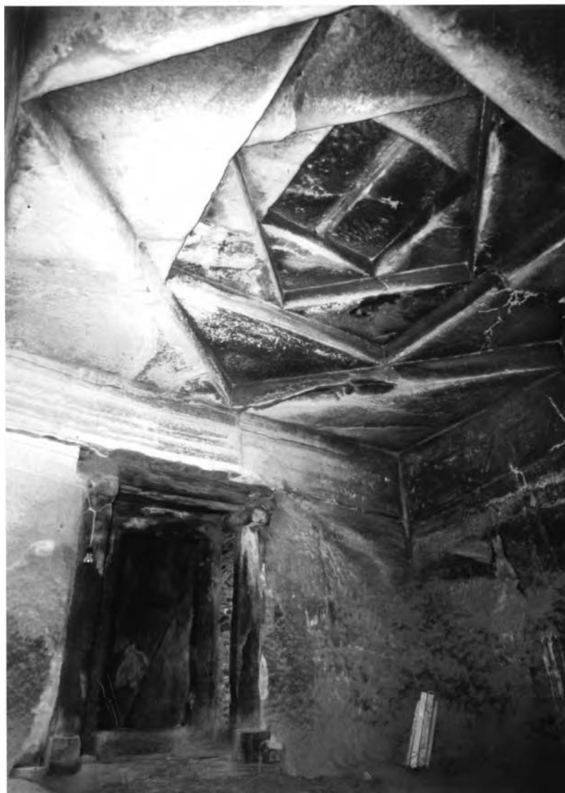
Fig. 81 The southeastern chamber of Yohannes Metmek Gazien church, showing the rock-hewn lantern ceiling and a wooden door-frame set into the rock
