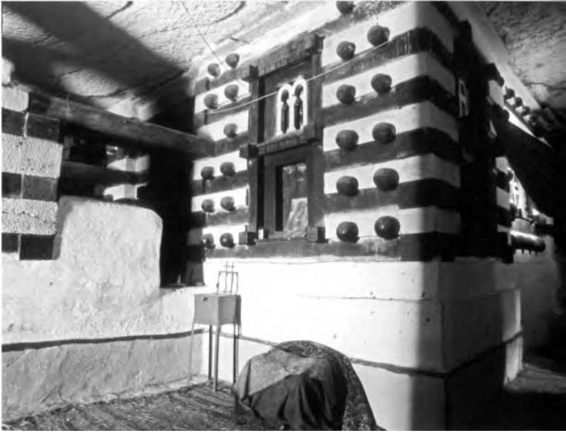
Fig. 82 The earliest component of the cave-set church of Mika'el Debra Selam, with decorative wooden beams-and-monkey-heads construction
