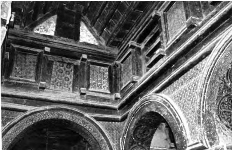
Fig. 92 Wooden construction of the nave at Imrahanna Kristos
