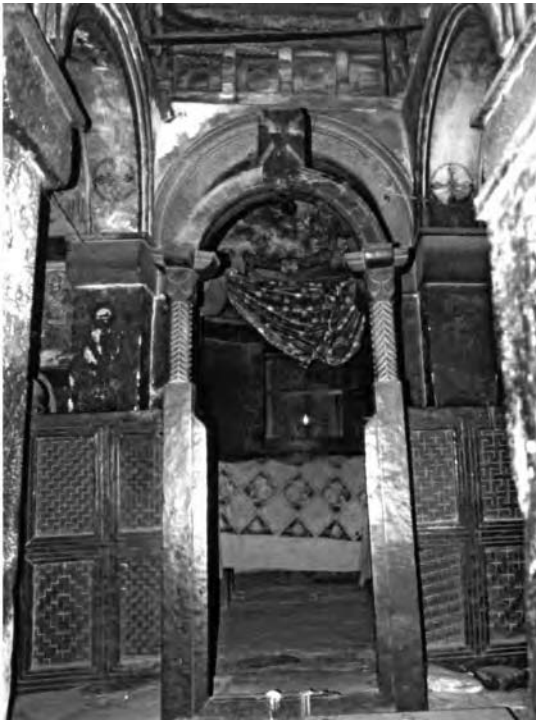
Fig. 82 The earliest component of the cave-set church of Mika'el Debra Selam, with decorative wooden beams-and-monkey-heads construction
