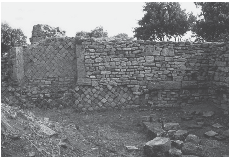
10.9. Roman bath in the agora with wall of opus reticulatum , looking south. Photo by William Aylward for the Troy Excavation Project.
