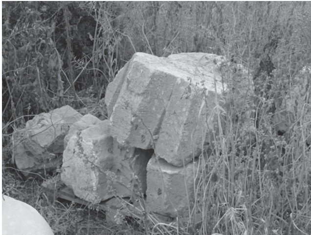
Fig. 21.12: Tas-de-charge (sandstone), broken, 3 concave ribs.
