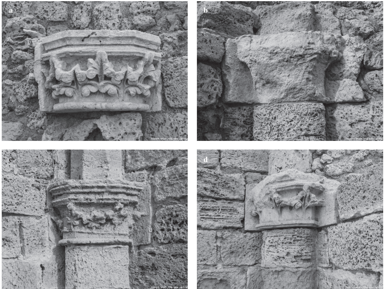
Fig. 21.4: a) Capital at south-east corner of GT1 ground floor: Limestone, fully preserved (photo: Assaf Peretz); b) Capital at south-west corner of GT1 ground floor: Sandstone, unpreserved face (photo: Assaf Peretz); c) Capital at north-west corner of GT1 ground floor: Sandstone, partly preserved (photo: Assaf Peretz); d) Capital at north-east corner of GT1 ground floor: Limestone, partly preserved (photo: Assaf Peretz).
