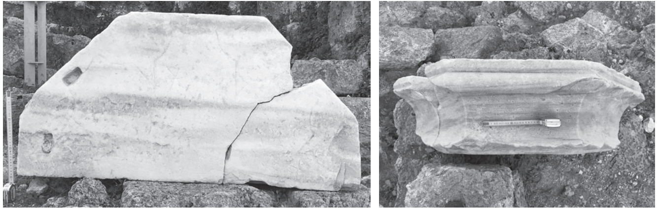
Fig. 21.33: Caesarea, half impost (115 × 69 cm) originally placed on octagonal pillar. Marks carved indicate the tripartite tas-de-charge of three complete concave ribs and a half on either side. Proconnesus Marble.
