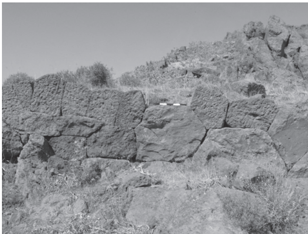
Fig. 1.4: Larisa East, eastern wall of the fort showing bed-rock, recessed toichobat , and the uppermost layer of wall base.
