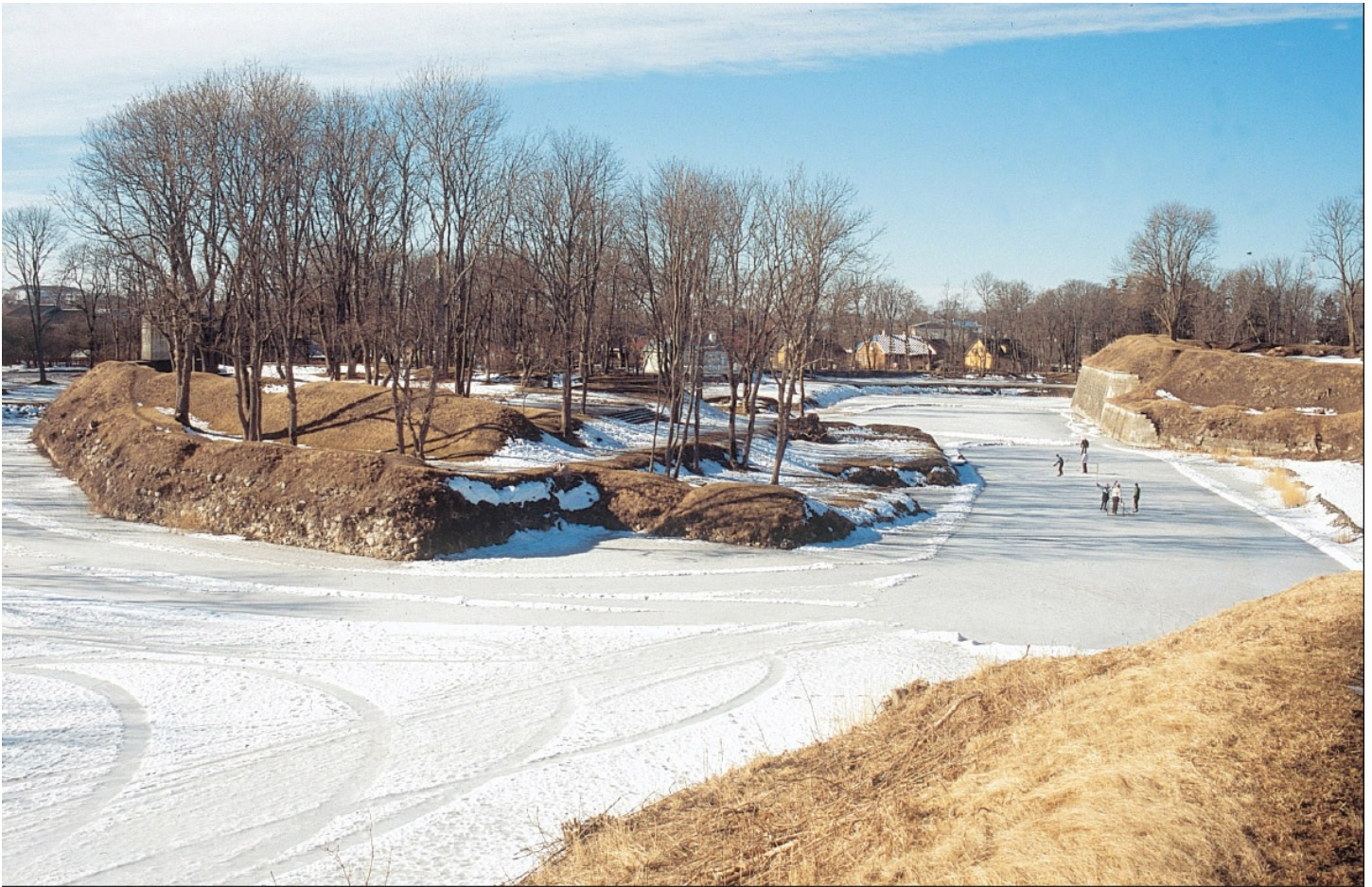
Plate 26 The snow and ice of winter show to great effect the shape and layout of a detached earthwork ravelin in the middle of the moat of Kuressaare Castle in Estonia. Contemporary Dutch examples are very similar in appearance
