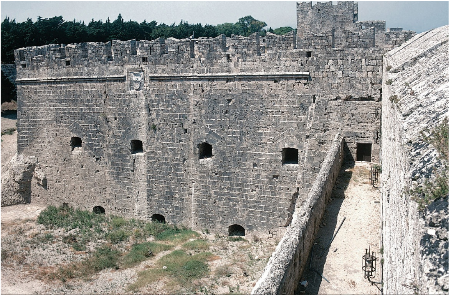
Plate 13 The Tower of St George in Rhodes, an early example of a pentagonal bastion that anticipated the angle bastion form. A near-vertical crack may be noted down the side. This was caused by a Turkish mine during the siege of 1522
