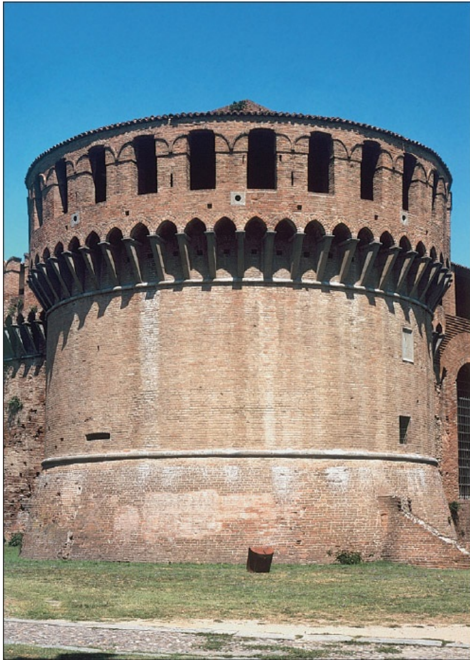
Plate 12 The rocca of Imola in Italy. In 1472 the existing rectangular corner towers were completely encased within the round towers in the rocca style that replaced them, and it is possible to walk round the inner tower within the outer one. This was a typical response to the challenge made by artillery to medieval fortification styles
