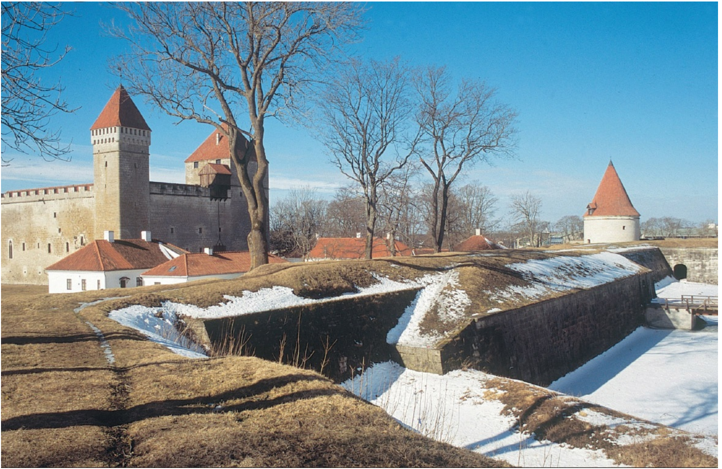
Plate 20 Three stages in the development of fortifications are shown in this view of the castle of Kuressaare, which lies on the island of Saaremaa in Estonia. To the left rear we have the very solid and tall medieval castle of the Livonian Order. To the right rear is a circular artillery tower dating from the late fifteenth century. The photograph is taken from one edge of a series of angle bastions that enclose the fortress
